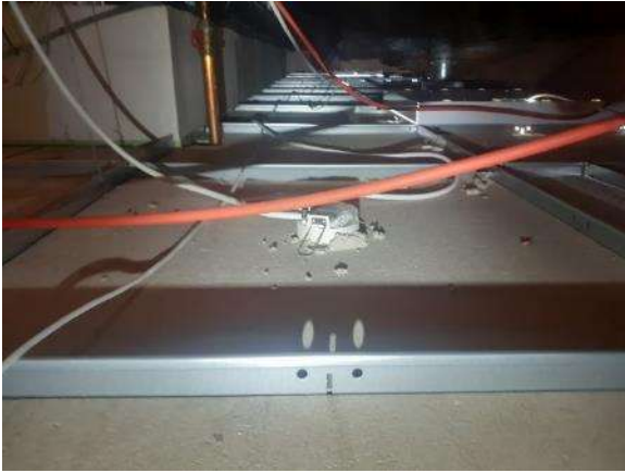
Photo 5 Roof void, showing no bat signs
