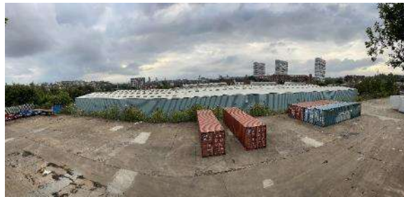
Photo 16 Hard standing vehicle and storage area from east
