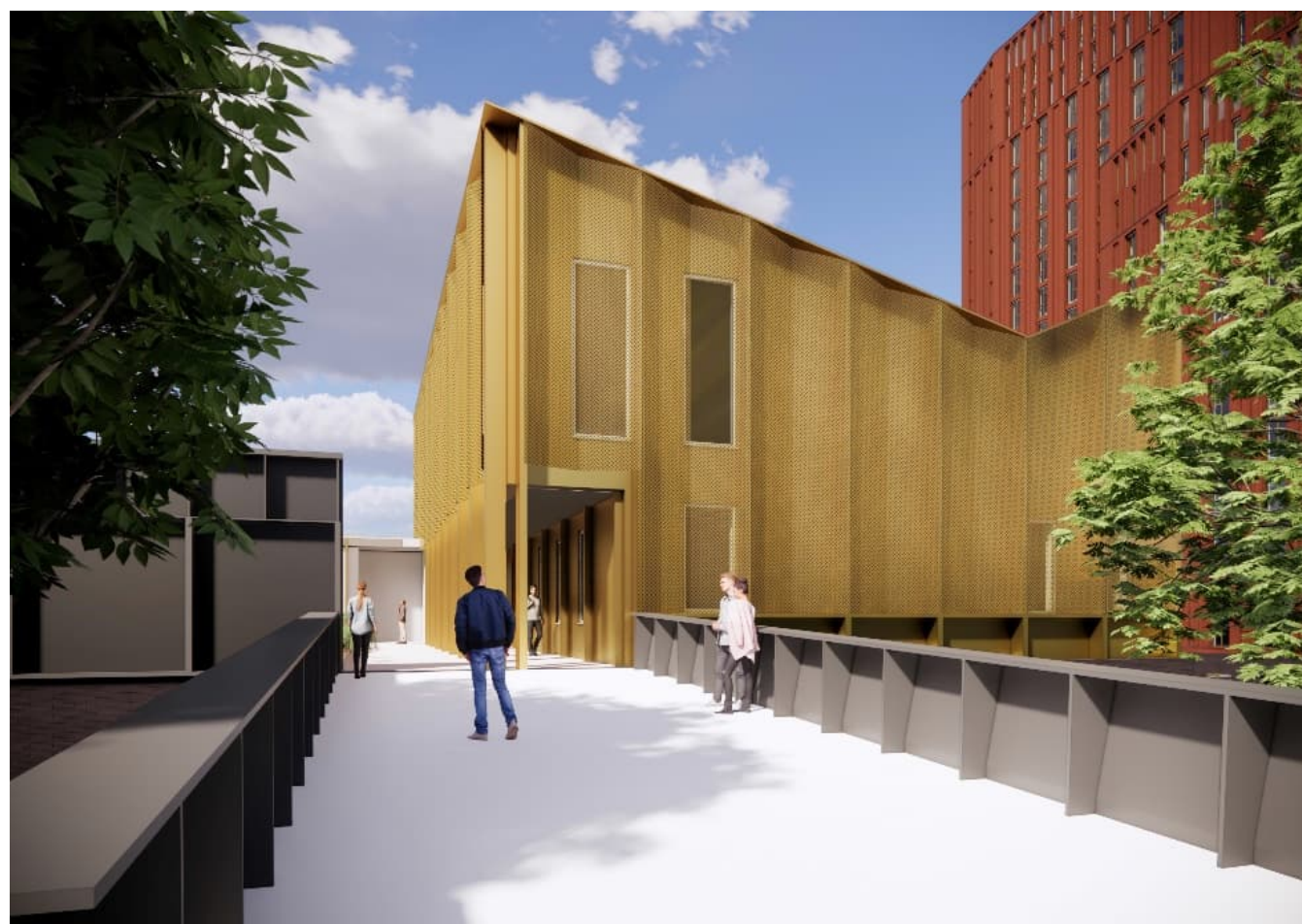
Figure 18 - Metal Mesh for Shading on SO Building
