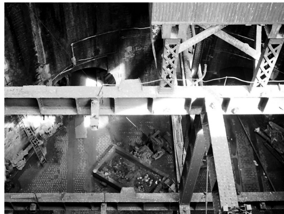
Image top: Technical Drawing of the Tunnel Under the River Clyde (1890) Image left: Rotunda Carriage Entrance (1896) Image right: Inside Rotunda Shaft (date unknown)
