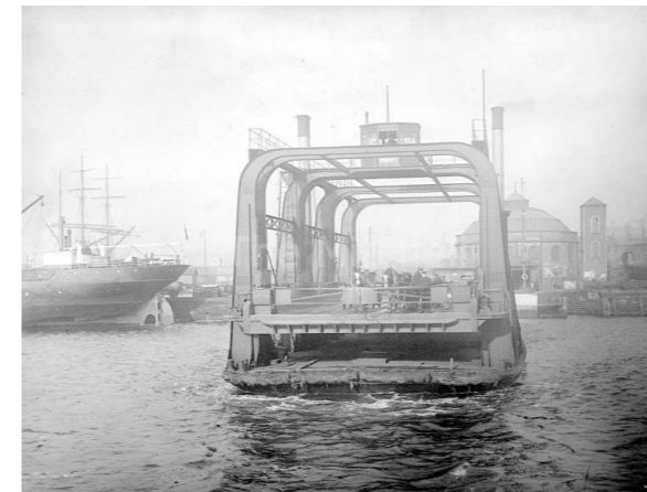
Figure 3.10 View of patent vehicular elevating ferry steamer with North Rotunda in the background 1914 CC Mitchell Library
