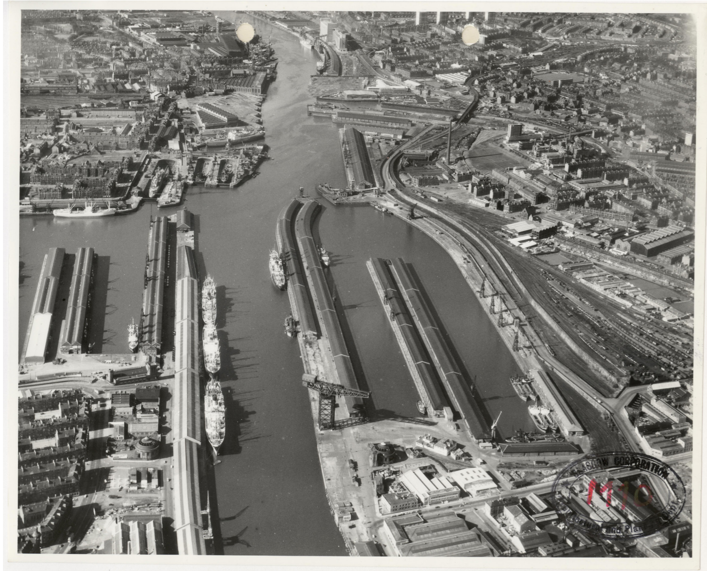
Figure 3.12 Aerial Photo looking west towards Queens Dock with Rotunda visible in the foreground. CC Glasgow City Council Planning Department 1966
