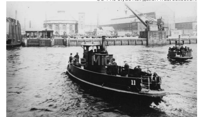
Figure 3.11 View of patent vehicular elevating ferry steamer with North Rotunda in the background 1914 CC Mitchell Library
