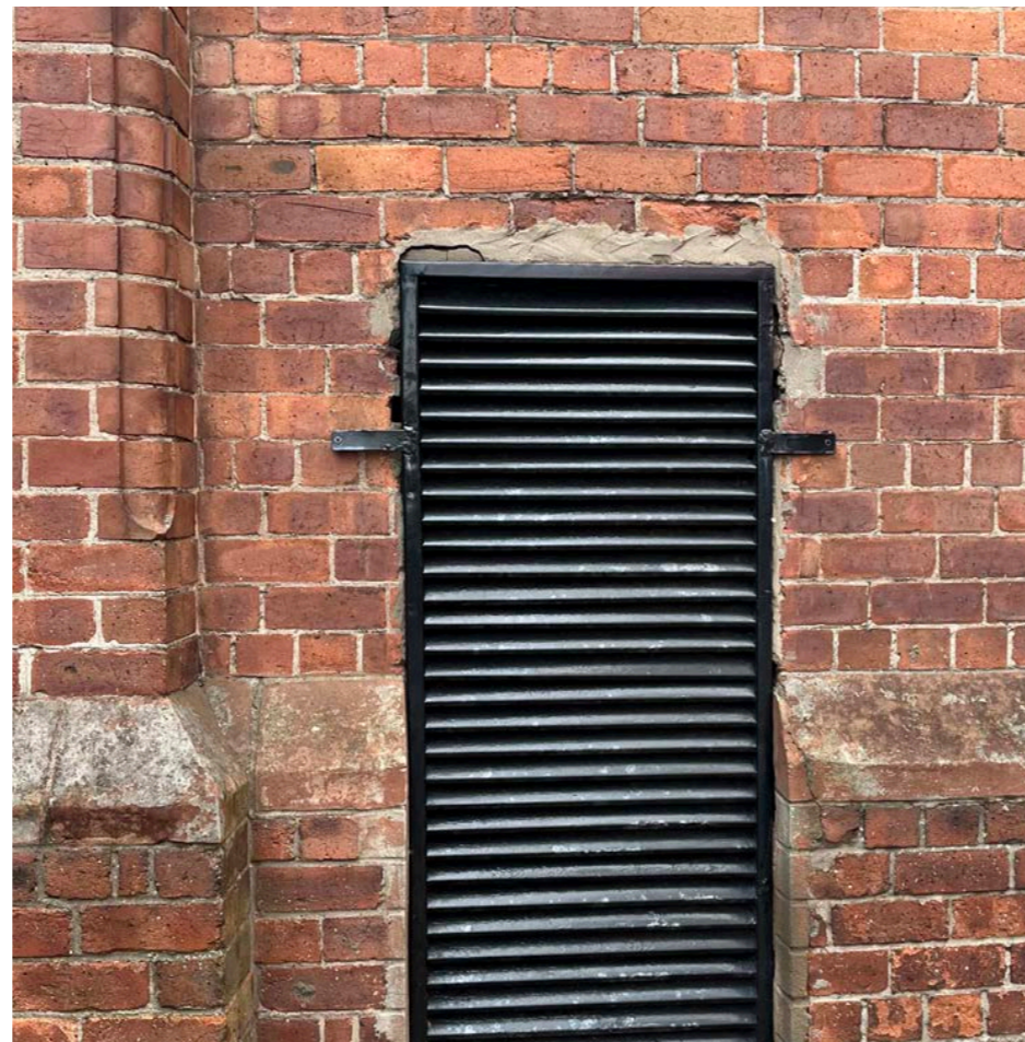
Image top left: existing cupola Image top right: existing roof slates Image bottom left: existing roof structure Image bottom right: existing brickwork & stonework
