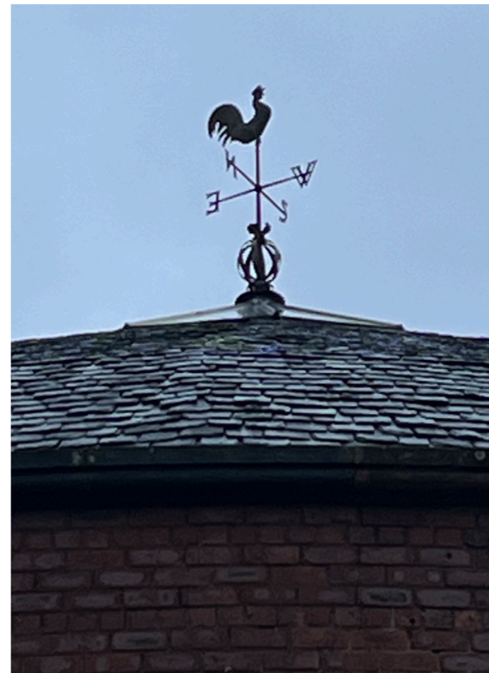
Image top left: aerial view of existing roof Image top right: existing service penetrations and standing water in gutters Image bottom left: general condition of existing roof Image bottom right: existing weathervane (assumed not original)
