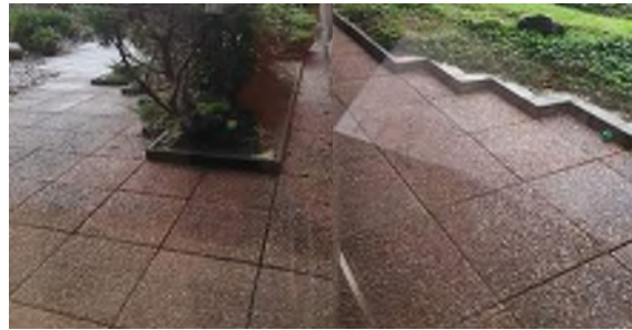
Figures 58 & 59 - Existing Concrete Paving Slabs
