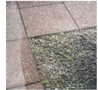
Figure 61 - Existing Gravel Strip
