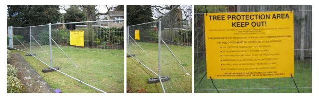
It may *in some cases* be acceptable (e.g. on smaller sites) for rubber or concrete 'feet' at the base of heras fencing to be pinned to the ground or for short outriggers to attached to the fencing and pinned to the ground in lieu of a full scaffold framework. As this is a relatively small domestic project this approach is considered appropriate in this instance.
