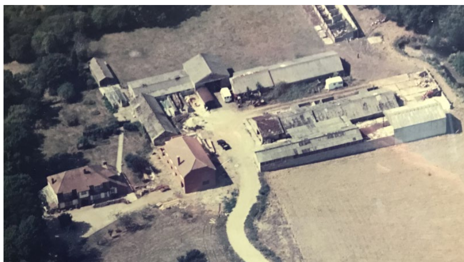
Figure 1 – Aerial photograph of site showing former extent of buildings.
