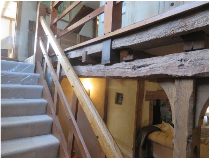
Stairs and balustrade to be removed
