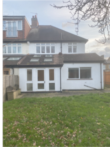
Rear Elevation Photo
