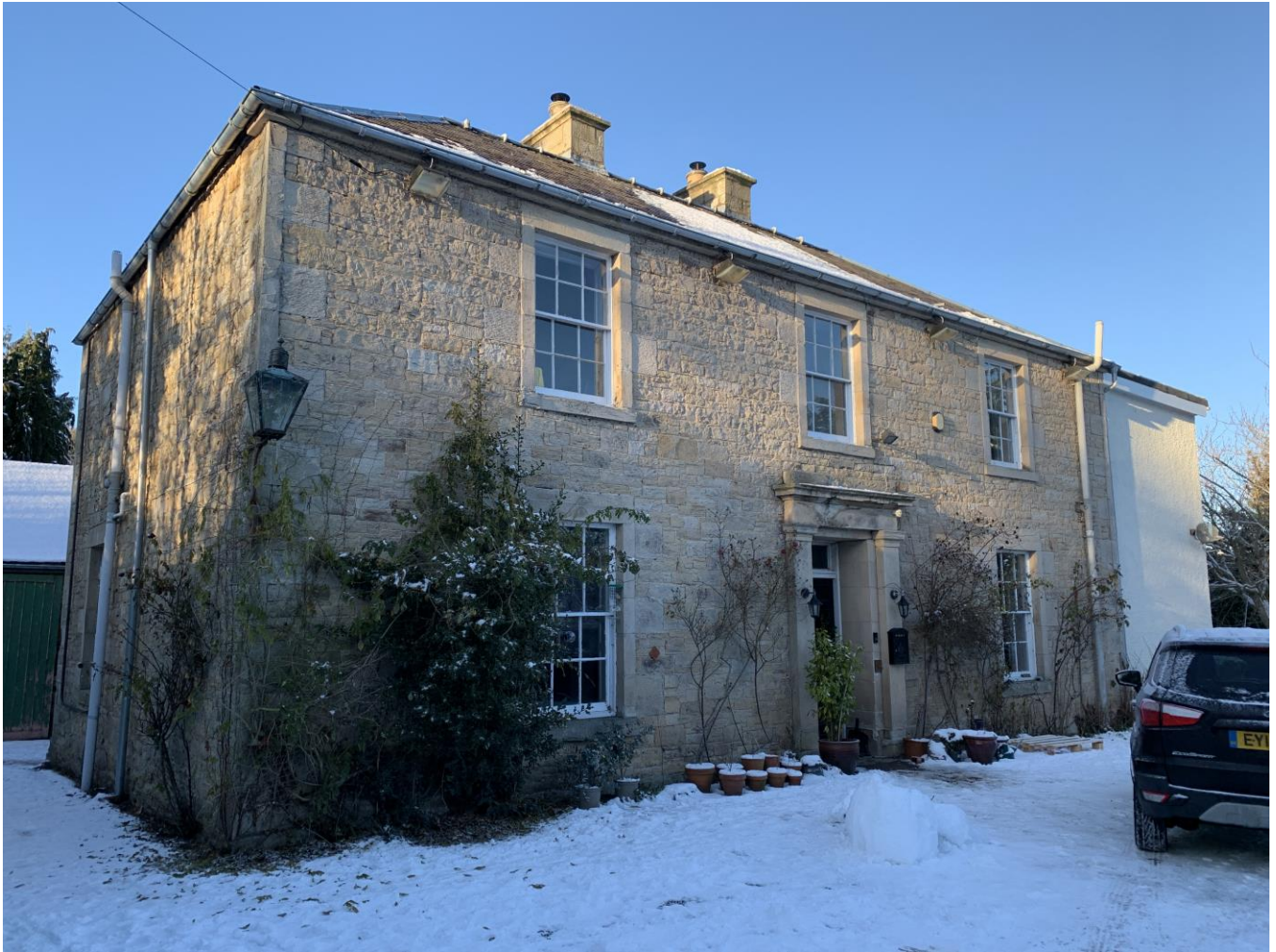
Front/SE Elevation (Viewed from South)
