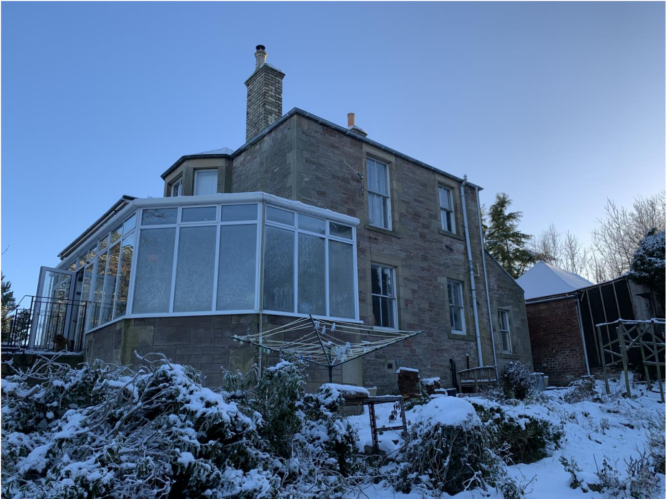
Rear/NW Elevation (Viewed from North)
