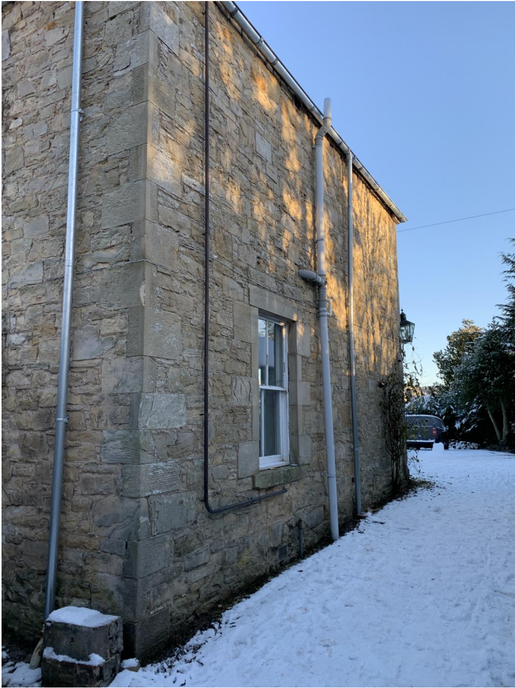
Side/SW Elevation (Viewed from West)
