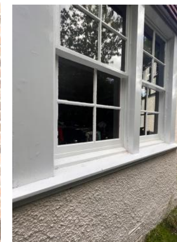
Timber frame sash and case 8 pane windows painted white to match existing
