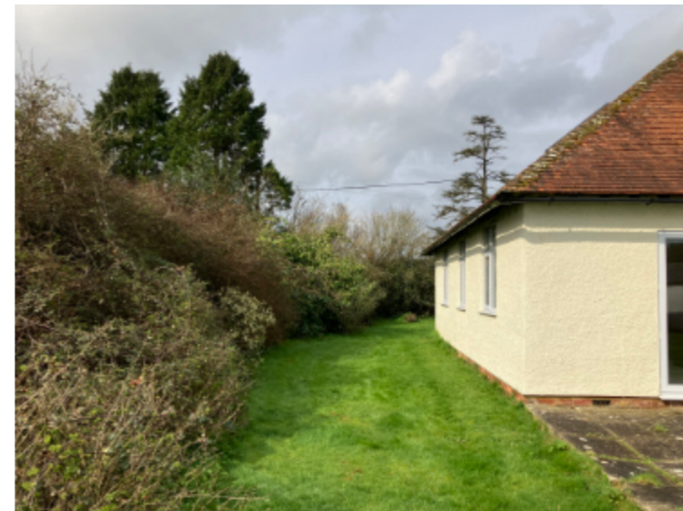
VIEW 05 - Looking West down the side of No.7.
