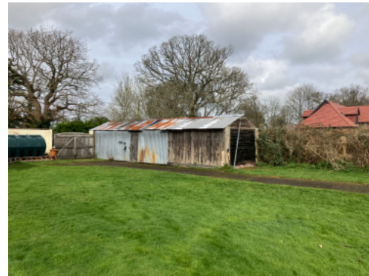
VIEW 12 - View North West looking at existing garage.
