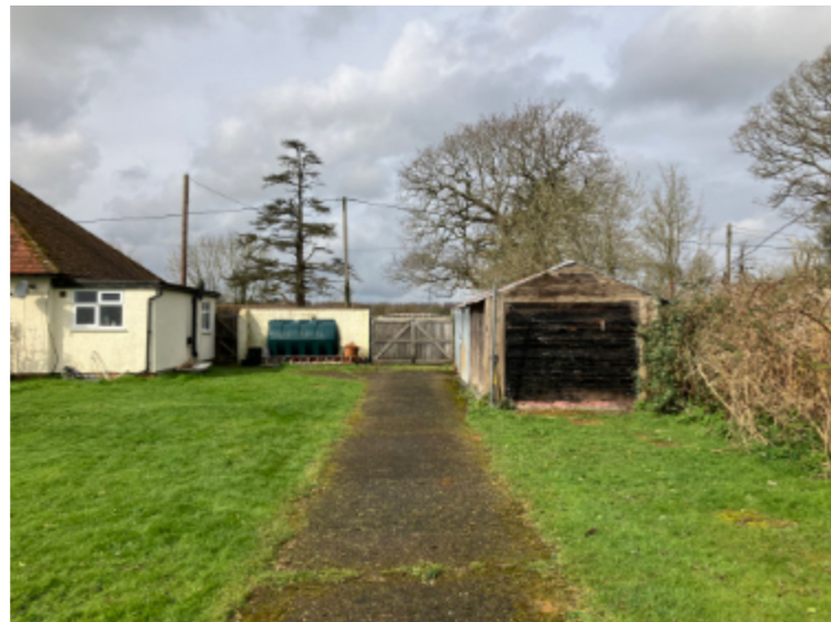
VIEW 04 - Looking West towards the garage.
