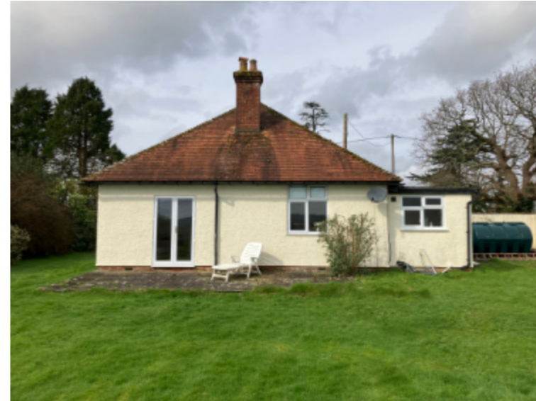
VIEW 02 - Looking West at the rear of no.7.
