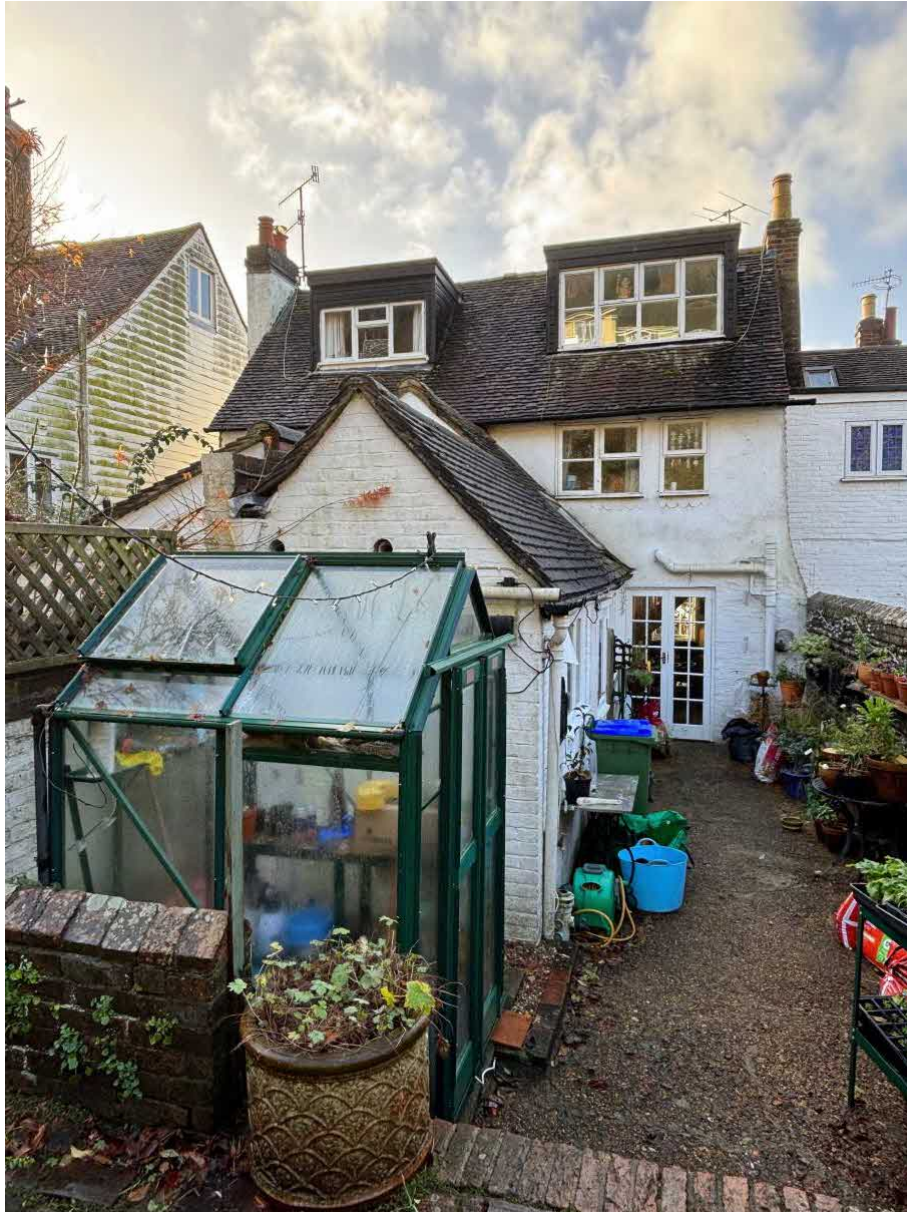
1. Rear elevation showing area of extension.
