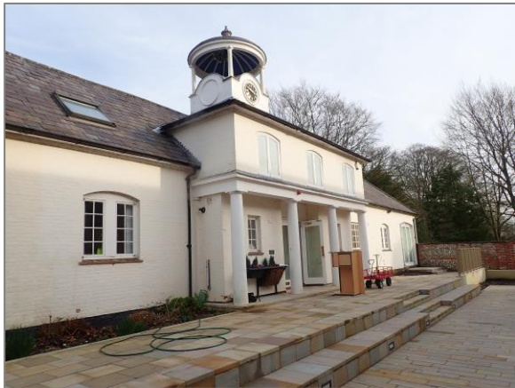
Photo 1 Front (south) elevation of Coach House
