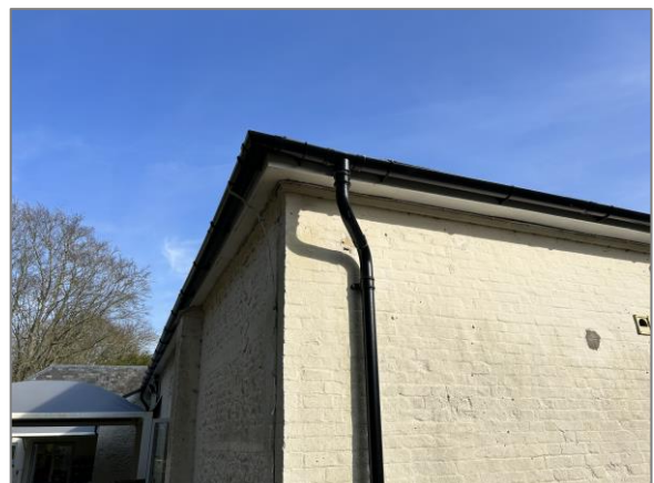
Photo 6 Existing building elevations where extension will tie in
