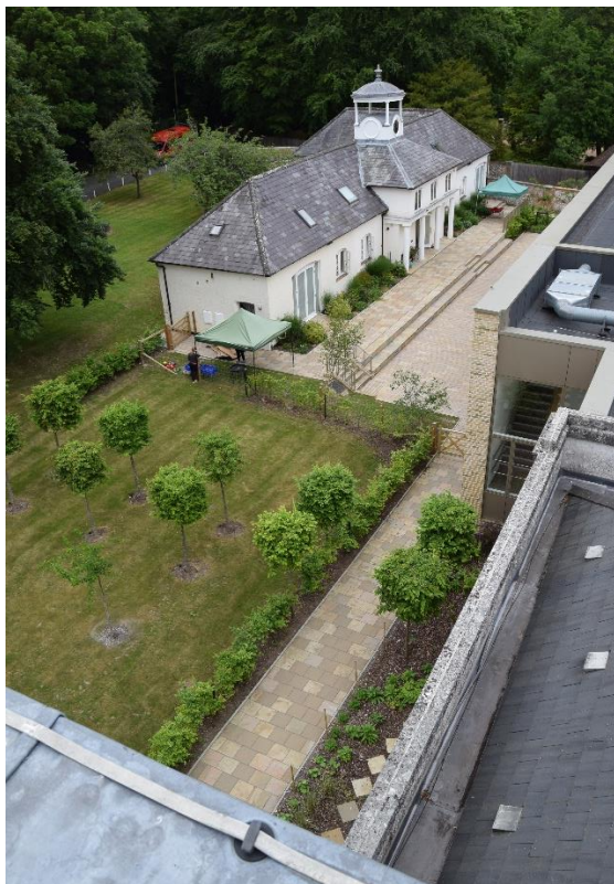
Looking north-west from roof of the main building towards the Coach House
