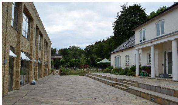
Looking west across courtyard; Coach House to the right
