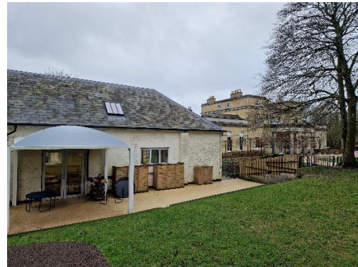
Rear elevation – northern façade
