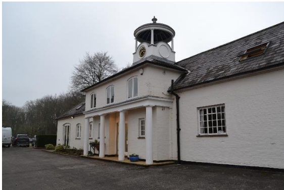
Frontage of building – southern façade
