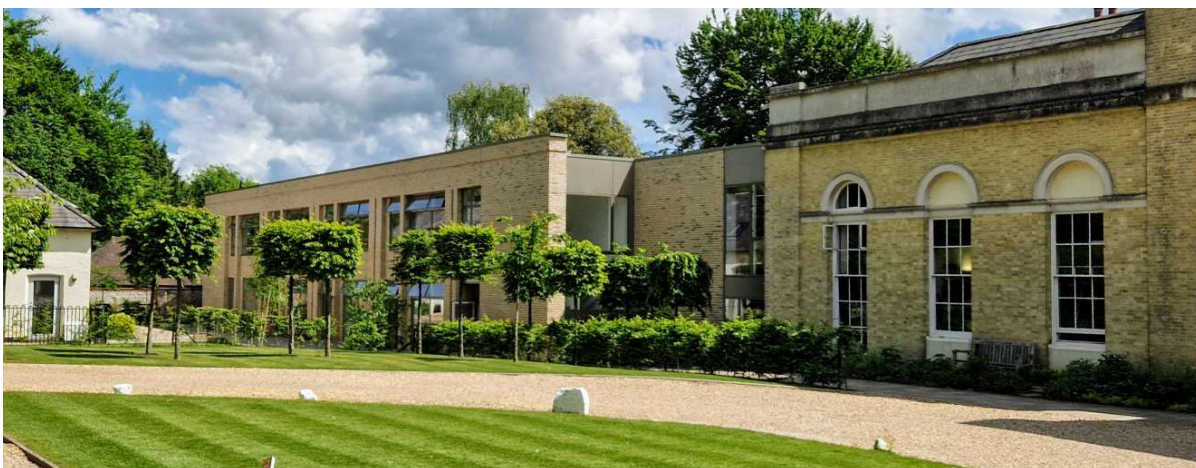
Recently completed extension
