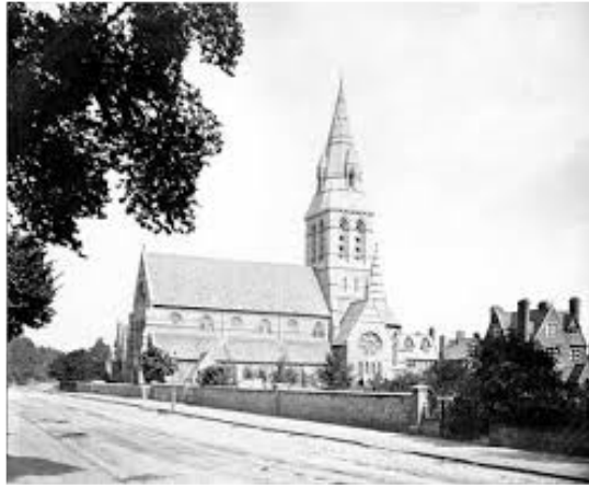
This image shows the completed church without trees along the Woodstock Road. The building in the foreground is the former vicarage.
