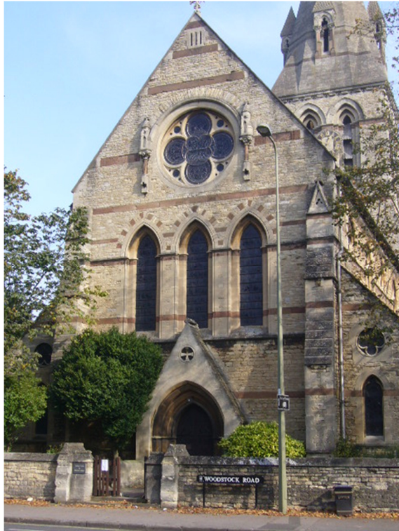
West elevation of St Philip and St James
