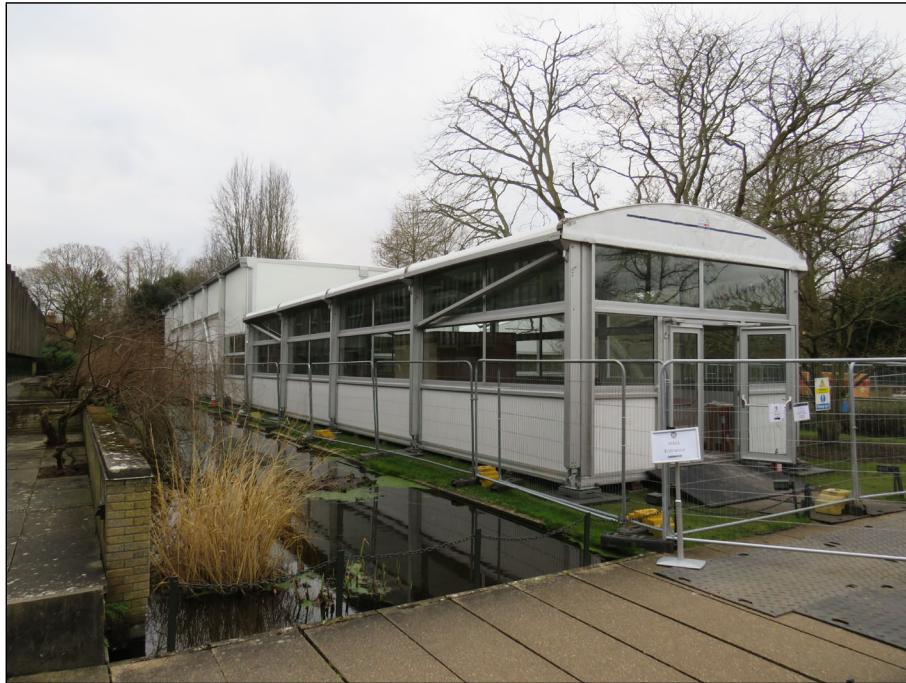
View 5 Looking south along eastern side of eastern Lecture Theatre Marquee
