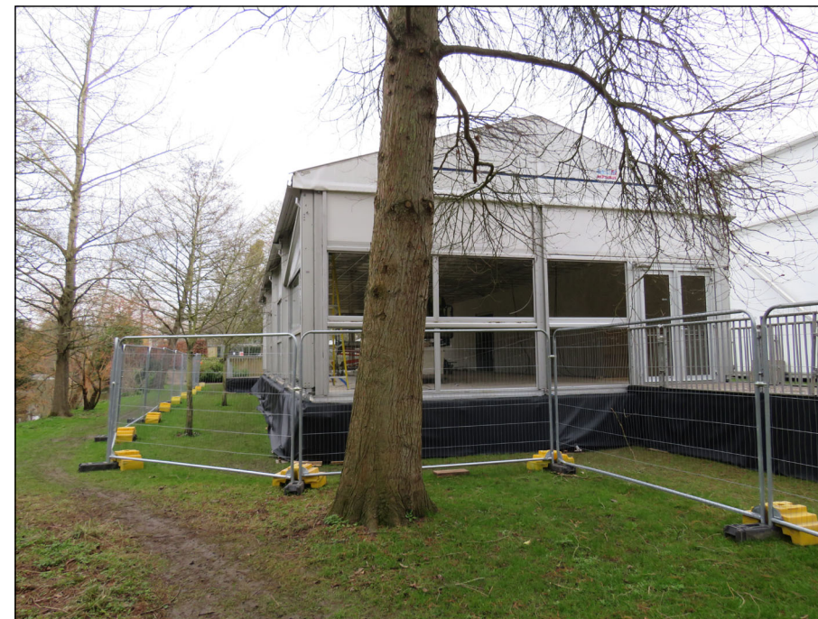
View 8 Looking north at south wall of western Lecture Theatre Marquee, with River Cherwell on left
