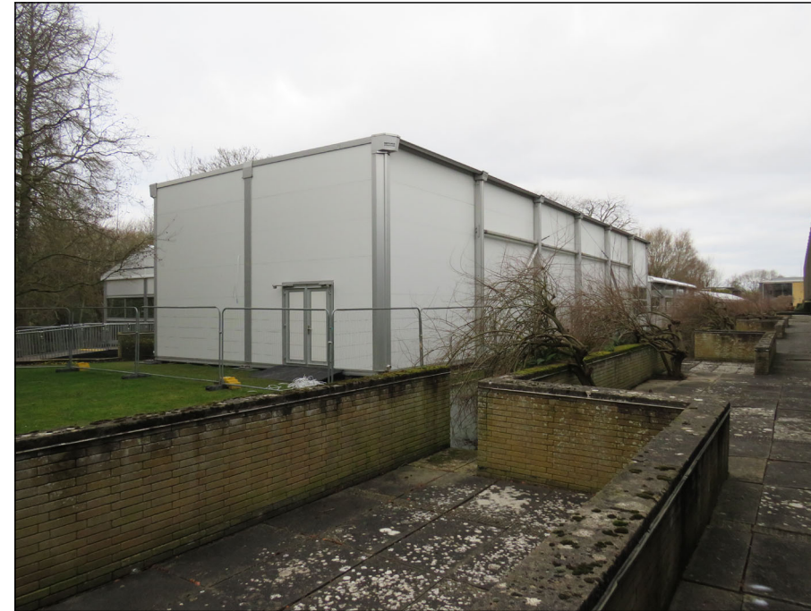
View 6 Looking north east at south wall of eastern Lecture Theatre Marquee
