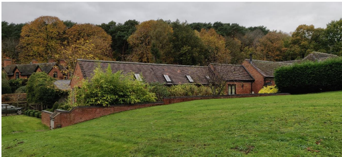
Fig 6. View of the building from the south east.
