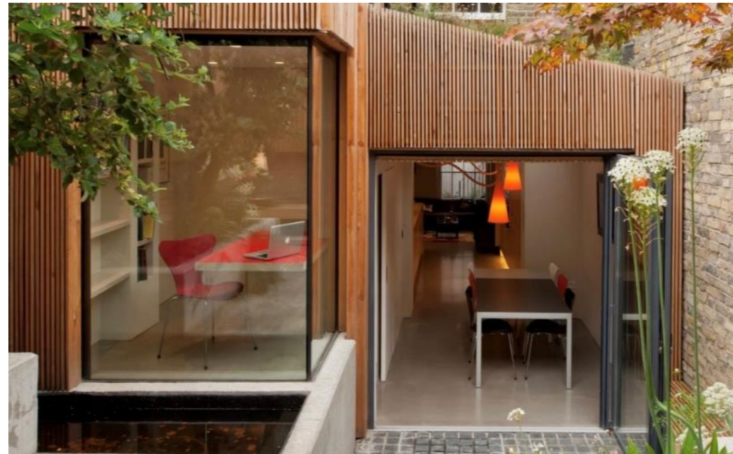
10. Image below showing timber cladding style
