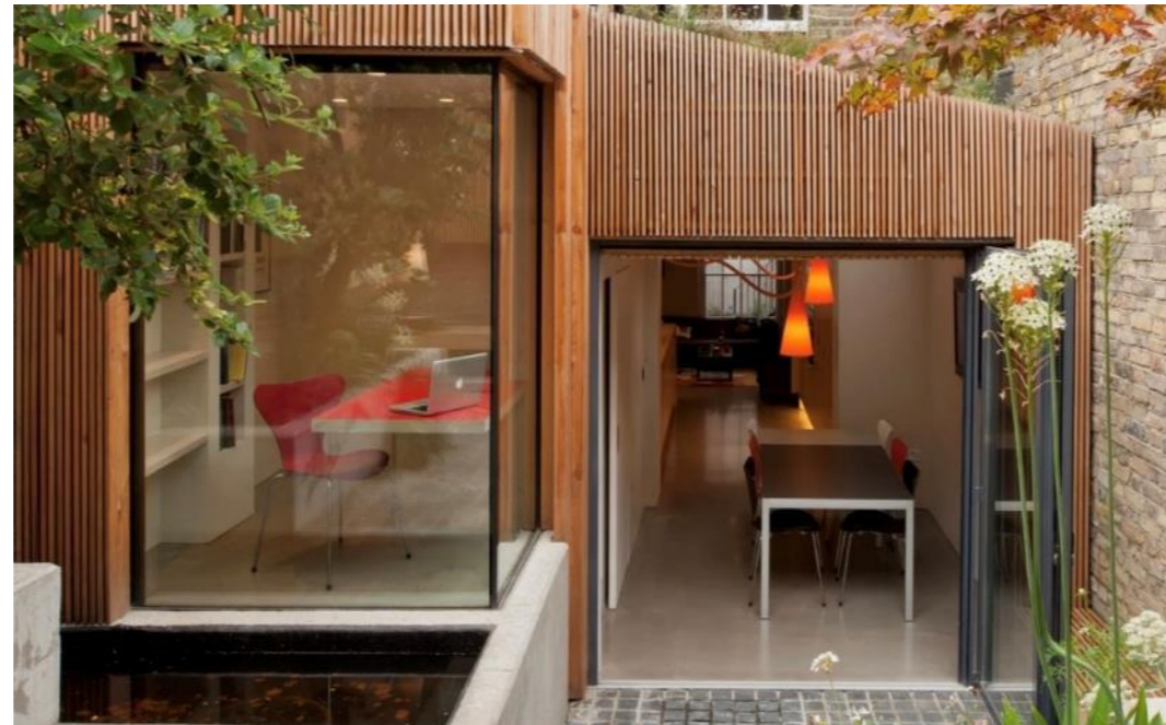
Image below showing timber cladding style
