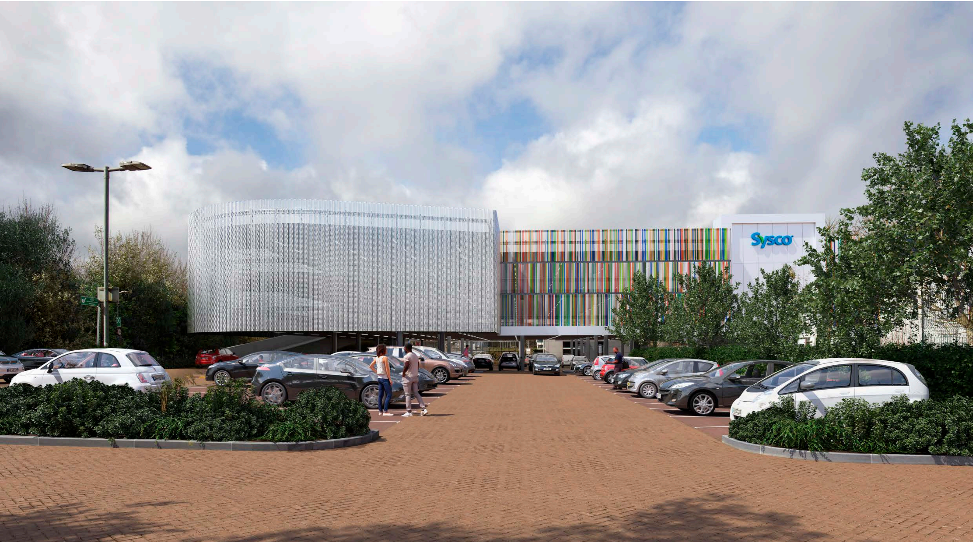
View west towards the office and multi-storey car park
