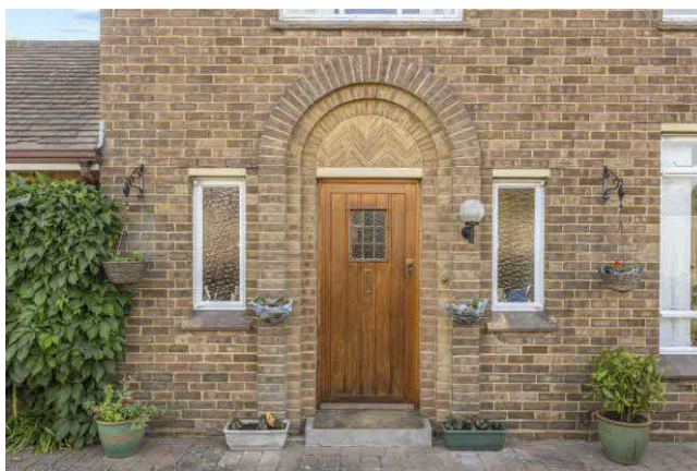
Brick detail over the front door retained.
