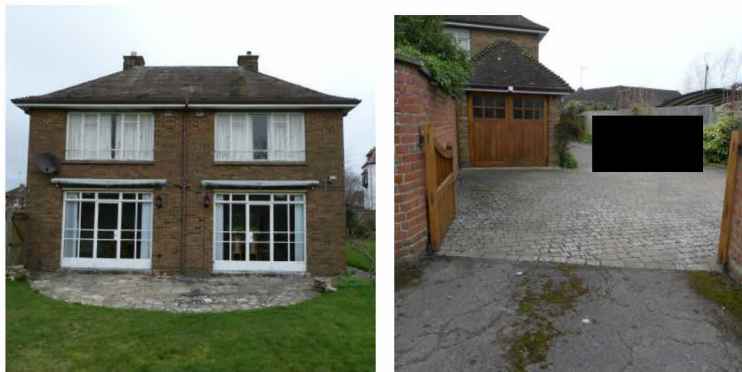
Left; South elevation of the dwelling to be extended. Right; Garage position and turning space from entrance.
