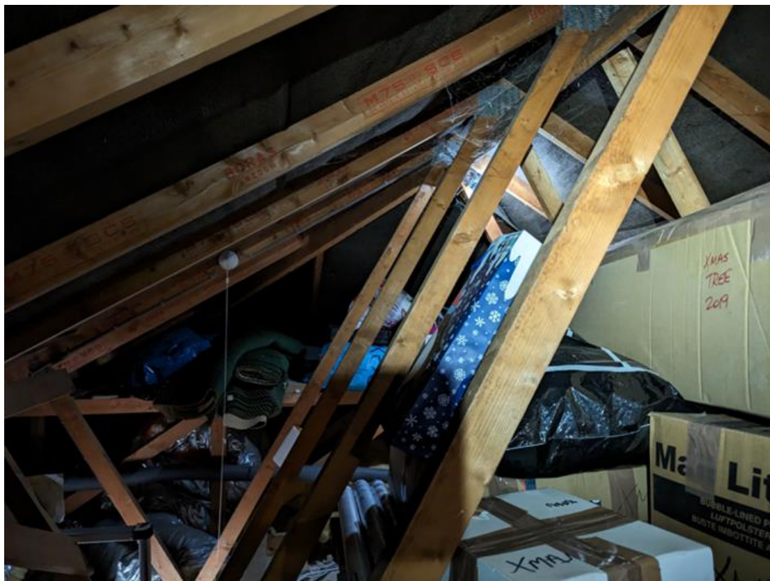
Photograph 5: The view of the loft space.
