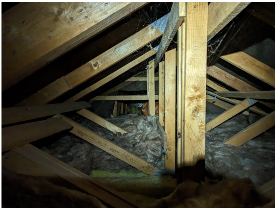
Photograph 4: The view of the loft space.
