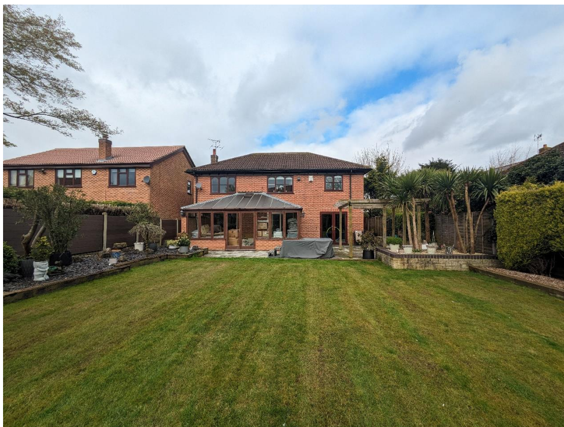
Photograph 2: The south east elevation of the building.
