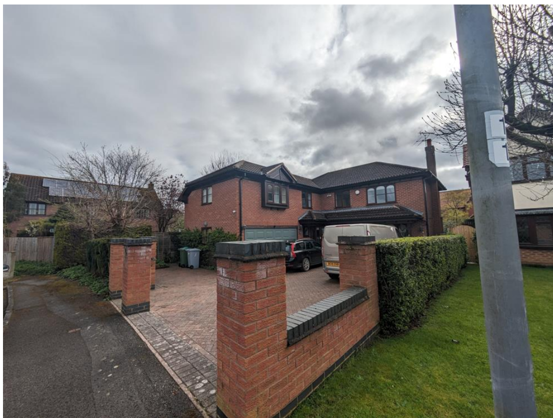
Photograph 1: The south and west elevations of the building.
