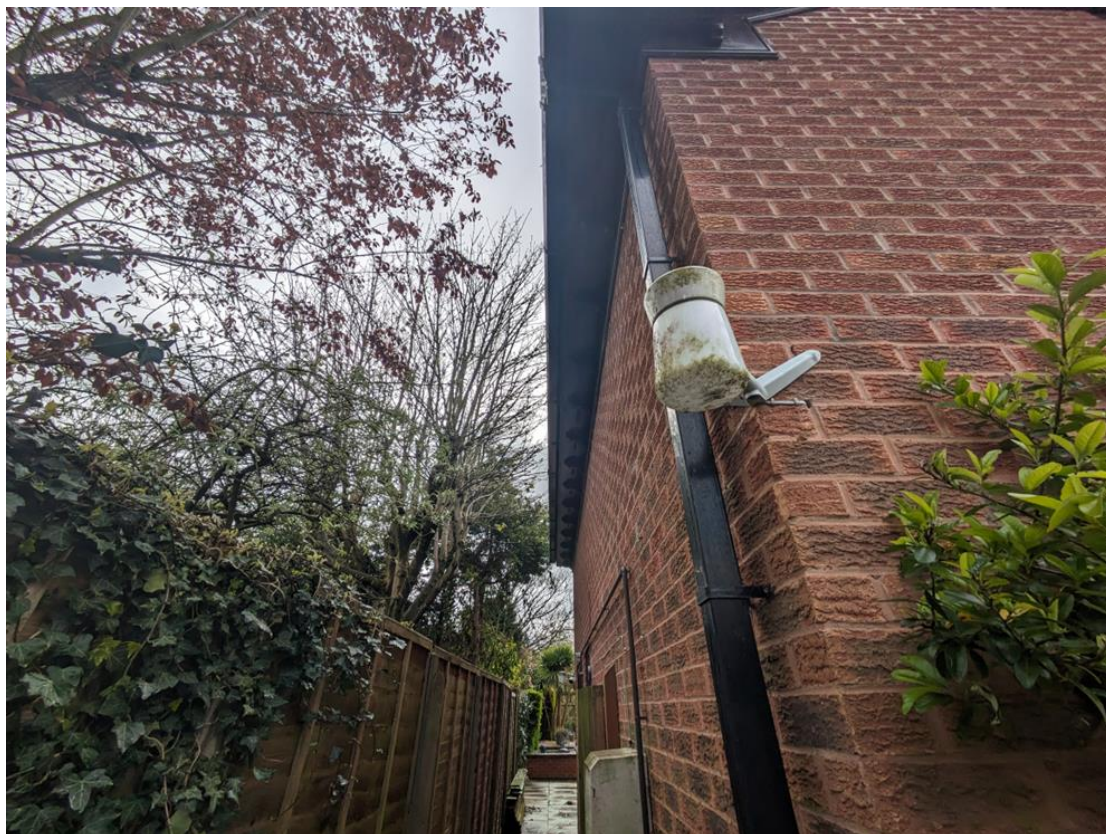
Photograph 3: The north elevation of the building.
