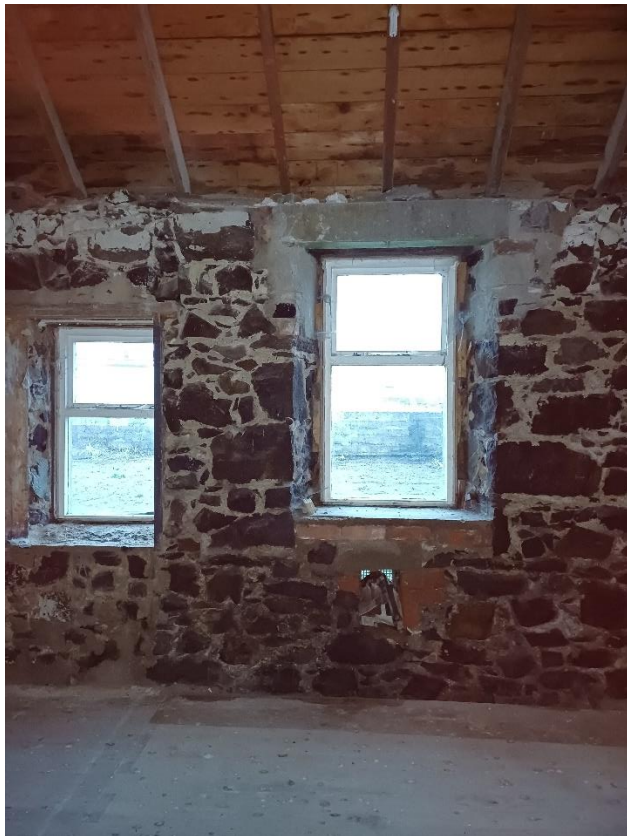
Existing window height to be used (Left window)
