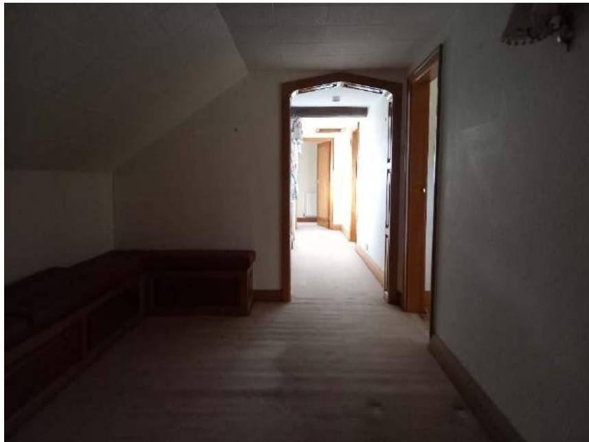
Plate 31: View looking north-west showing the first-floor corridor in the original part of the house. The doorway has been defined with modern panelling, but may respect an historic opening
