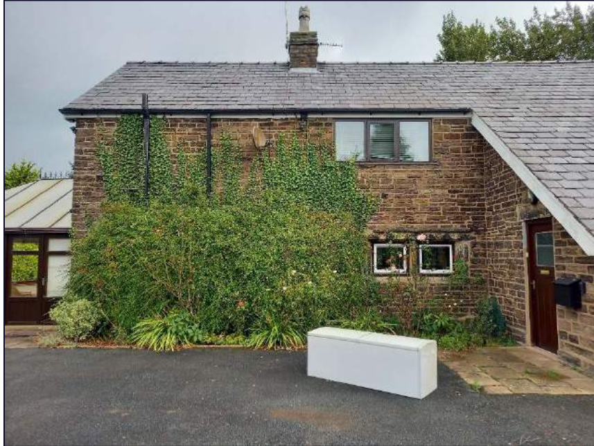
Plate 18: South-west elevation of the older section of Rotherham Top Farmhouse
