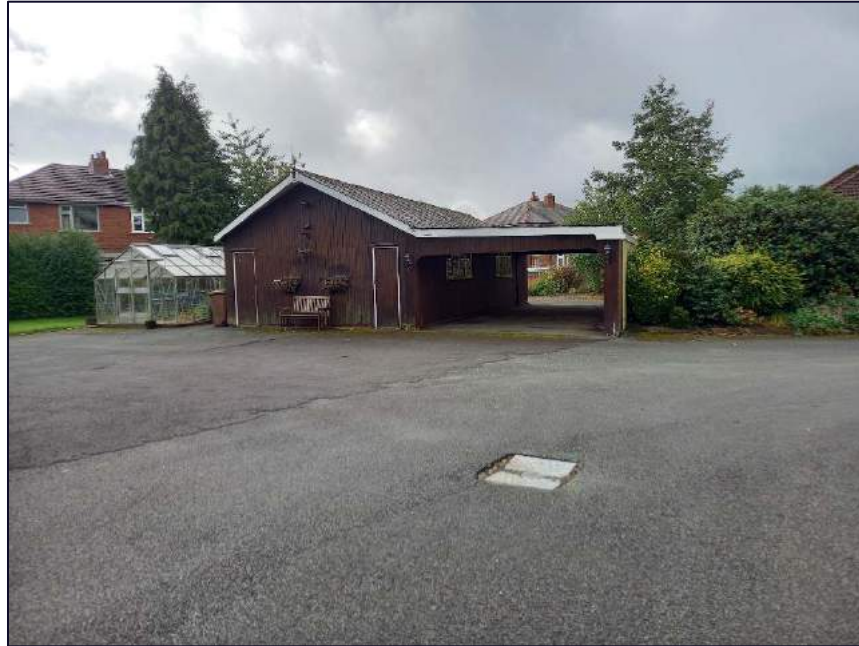
Plate 36: View looking south-west showing the wooden shed and car port to the west of the house
