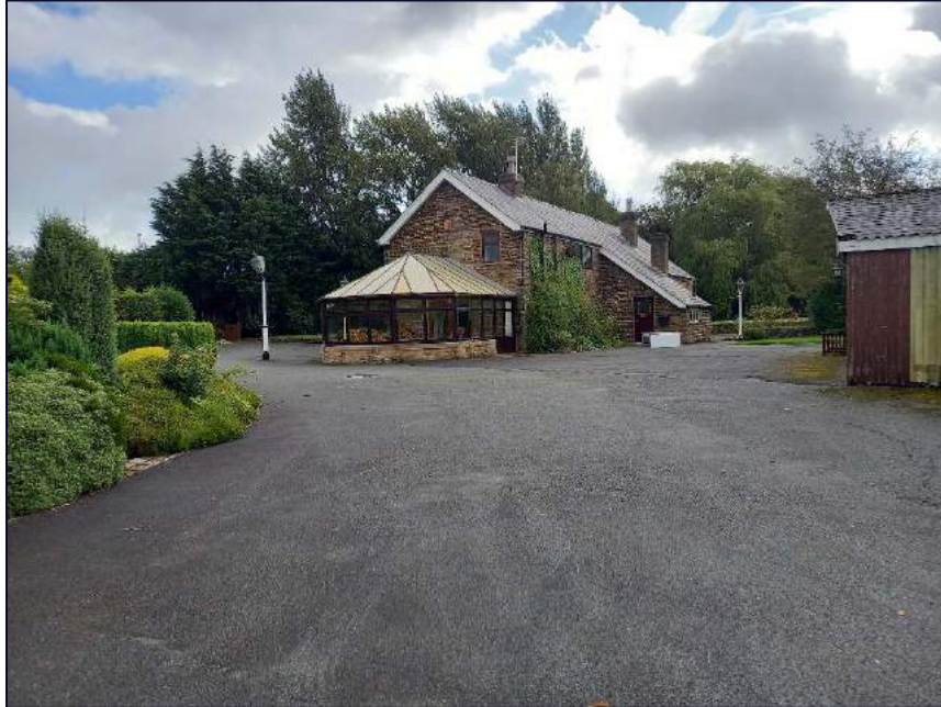
Plate 14: Rotherham Top Farmhouse as seen from the north-west of the site
