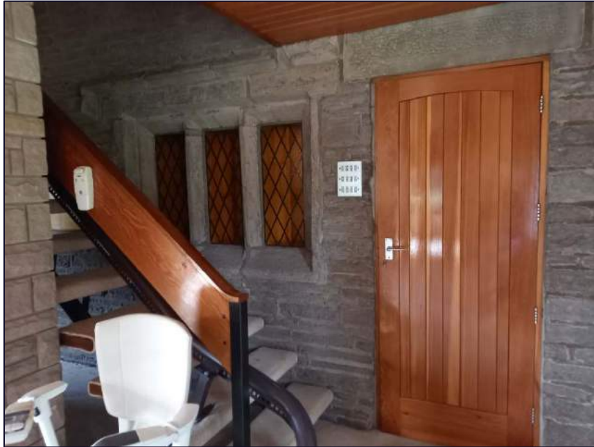
Plate 28: Original mullioned window which survives as a feature within the modern extension
