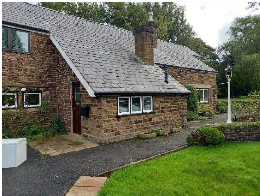
Plate 19: South-west elevation showing modern outshut partly utilising older stonework
