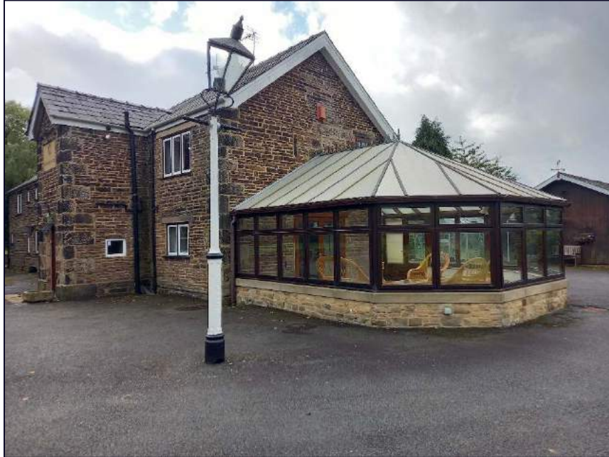
Plate 16: North-west elevation of Rotherham Top Farm with modern conservatory
