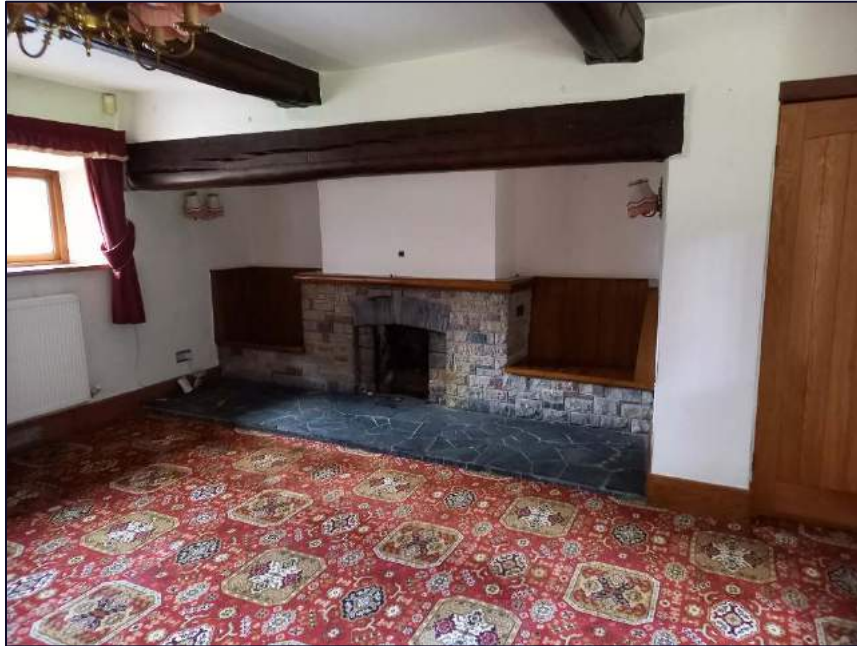
Plate 22: View looking north-west showing the large inglenook fireplace with modern fireplace, and moulded bressummer, ground floor of the original house
