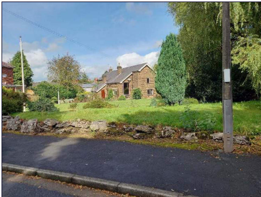
Plate 7: View looking north from Lea Road showing Rotherham Top Farmhouse and its associated garden
