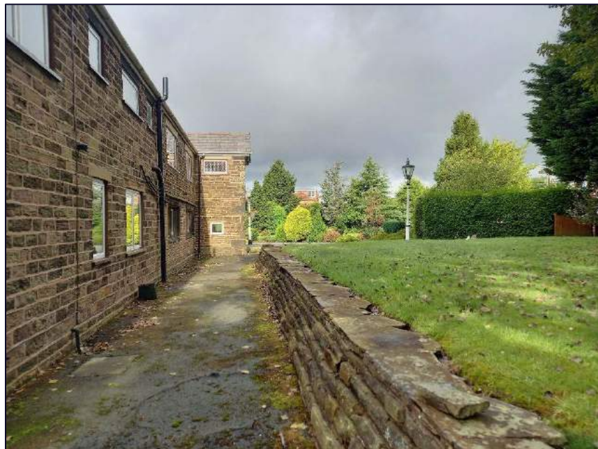
Plate 11: View looking north-west along the north-east elevation showing the projecting two-storey porch
