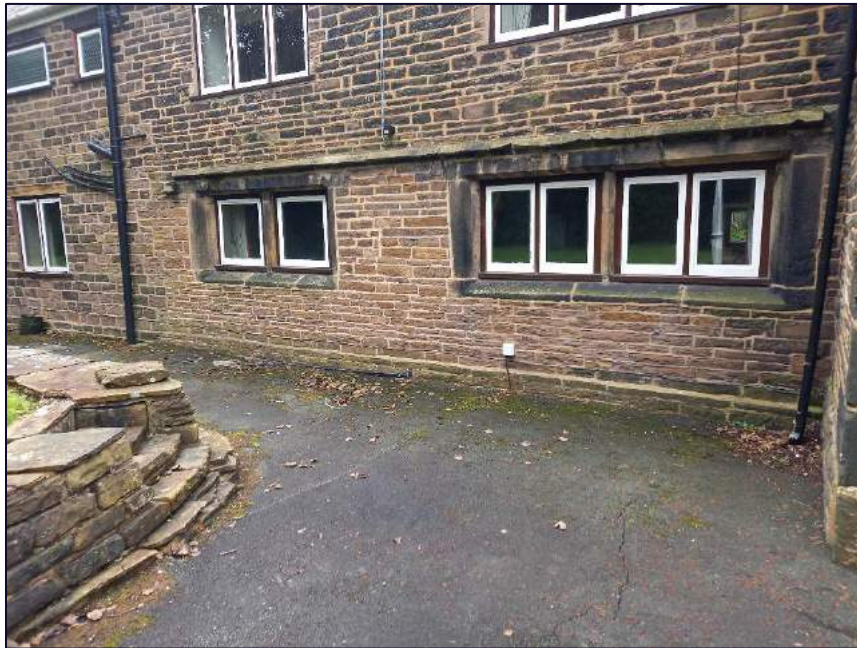
Plate 12: North-east elevation of Rotherham Top Farmhouse showing the ground floor windows with continuous hoodmould
