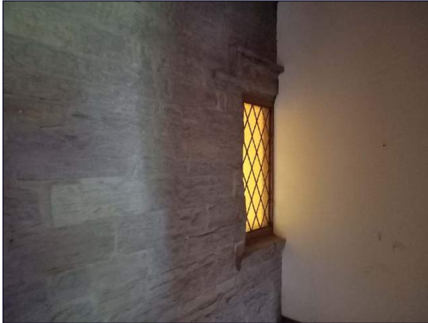
Plate 30: Part of a former two-light window in the original south-east elevation of the house, now incorporated but truncated within the modern extension
