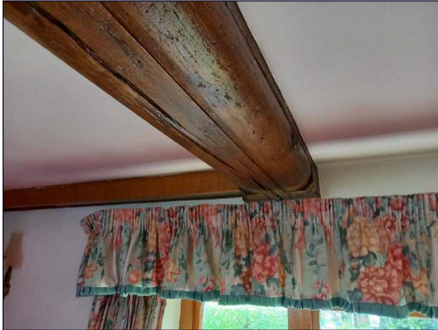
Plate 32: View looking south-west showing one of the exposed ovolo-moulded beams on the first floor
