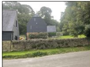
A - Existing Retained Stone Wall
