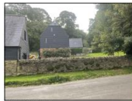
A - Existing Retained Stone Wall
