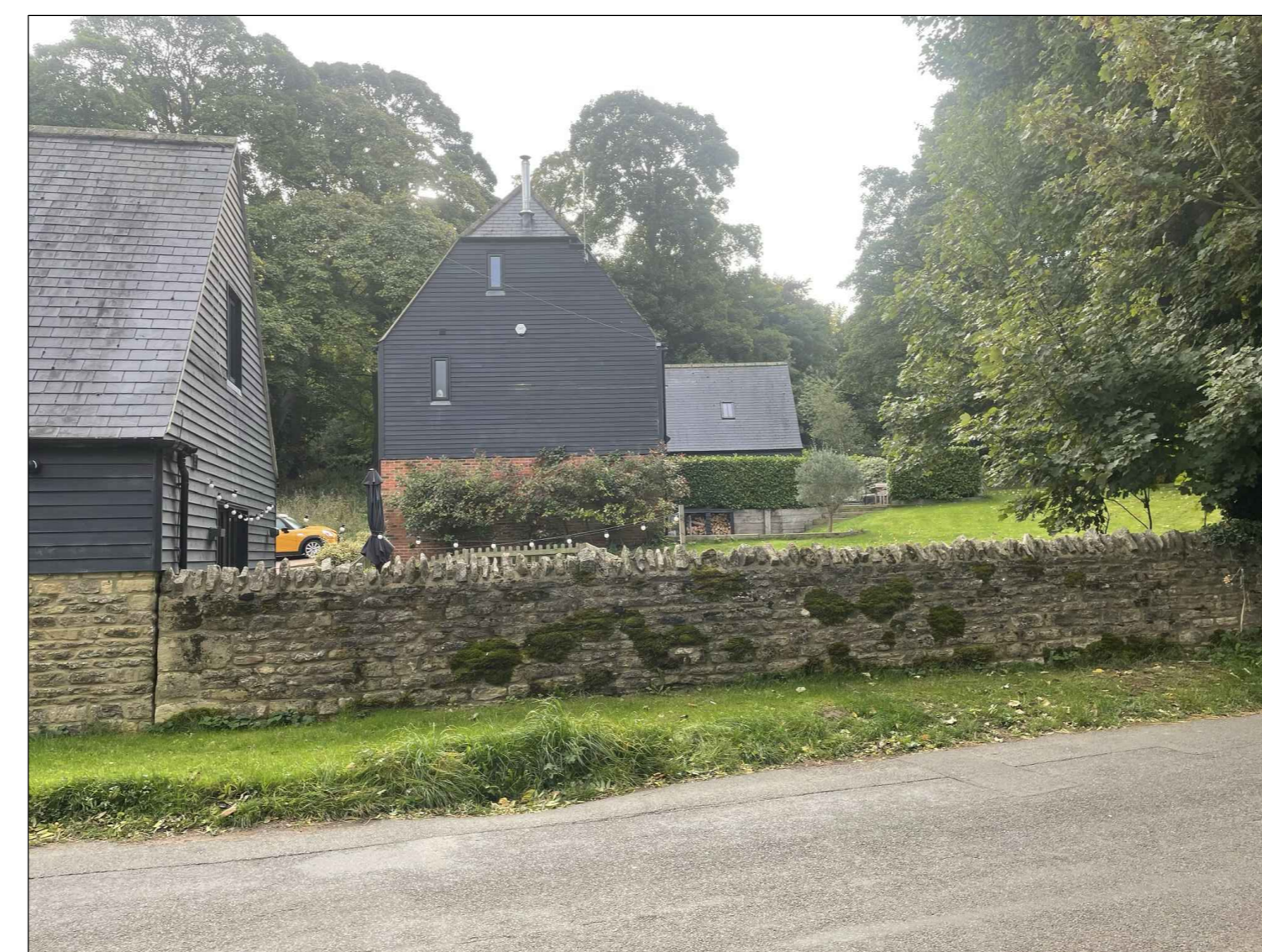
A - Existing Retained Stone Wall
