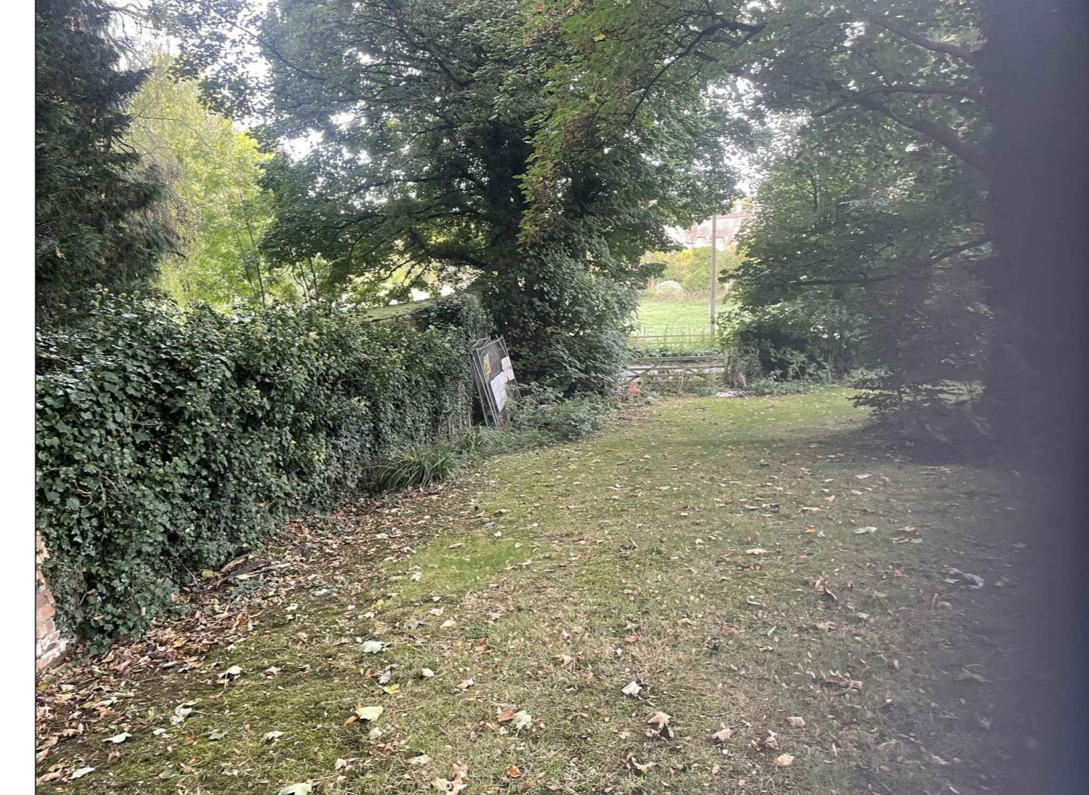
D - Existing Retained Brick Wall
