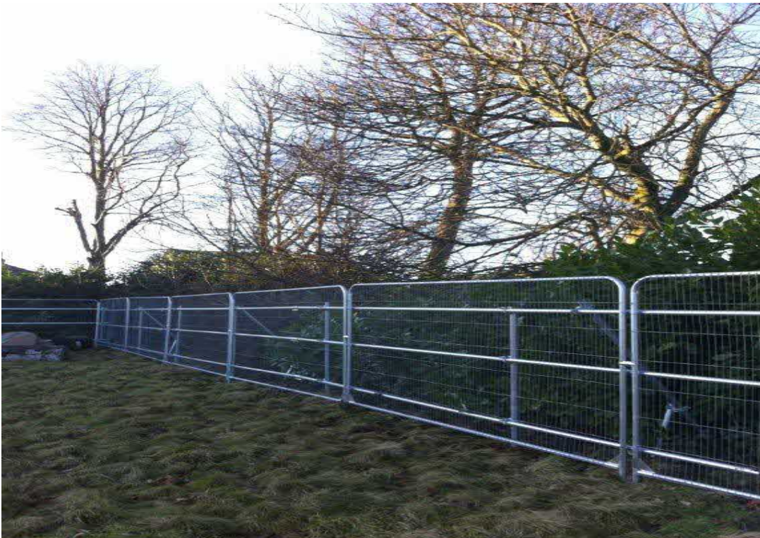
Figure 1 Photograph 1. Example of BS5837:2012 Tree Protective Fencing
