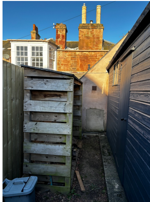
4. VIEW TOWARDS HOUSE AT SHARED BOUNDARY WITH 2 MARINE TERRACE
