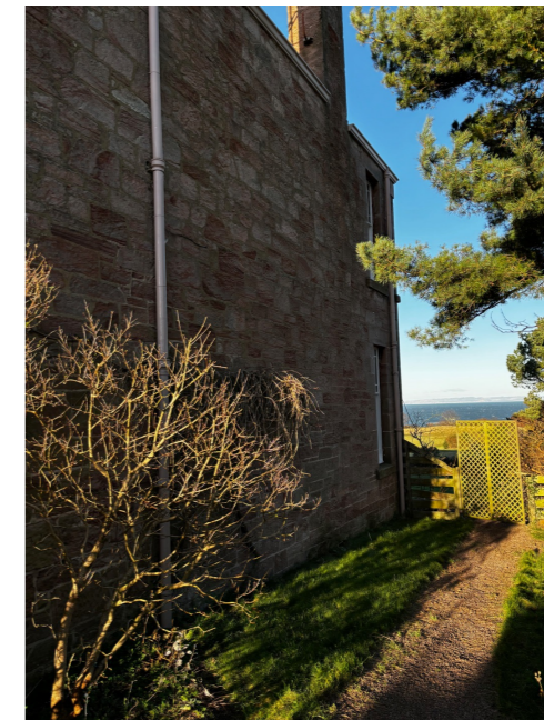
3. VIEW FROM SIDE GARDEN LOOKING TOWARDS GULLANE BENTS
