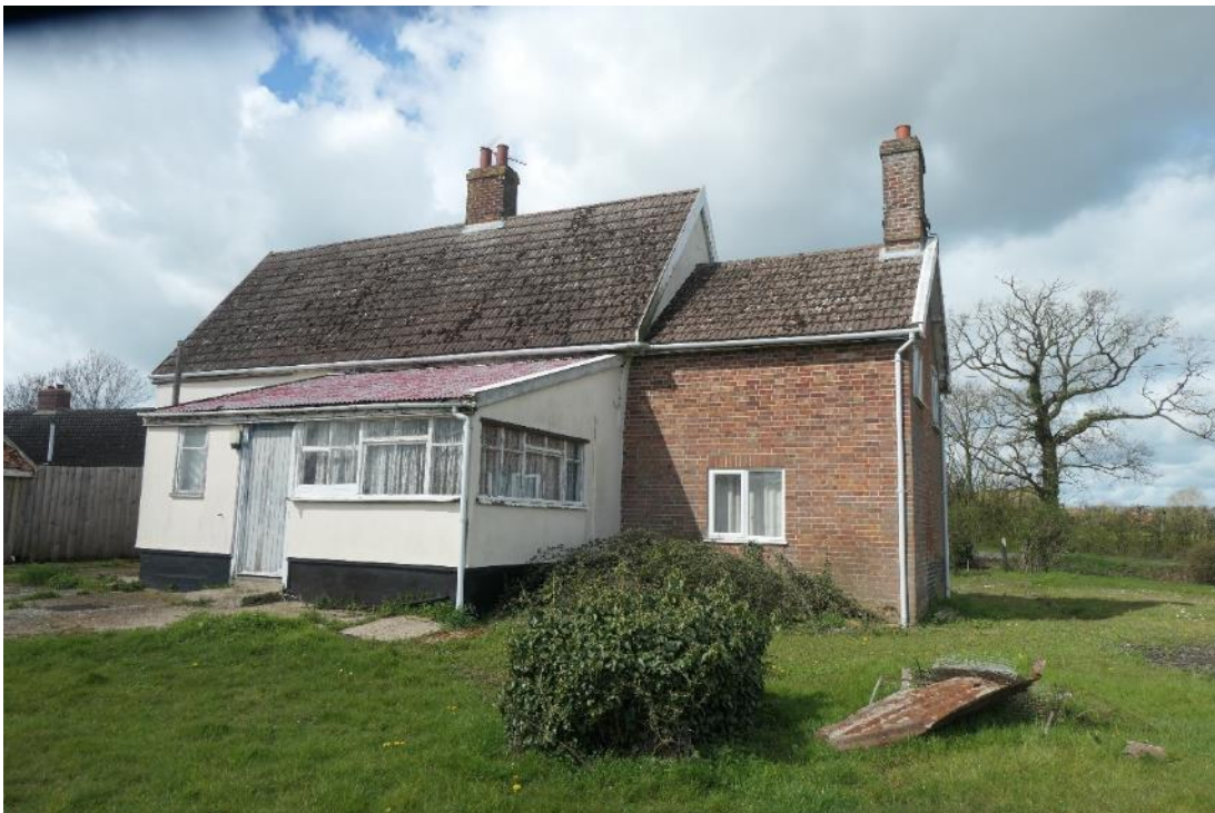
Photo 9 , north and east aspects of the building, looking southwest.
