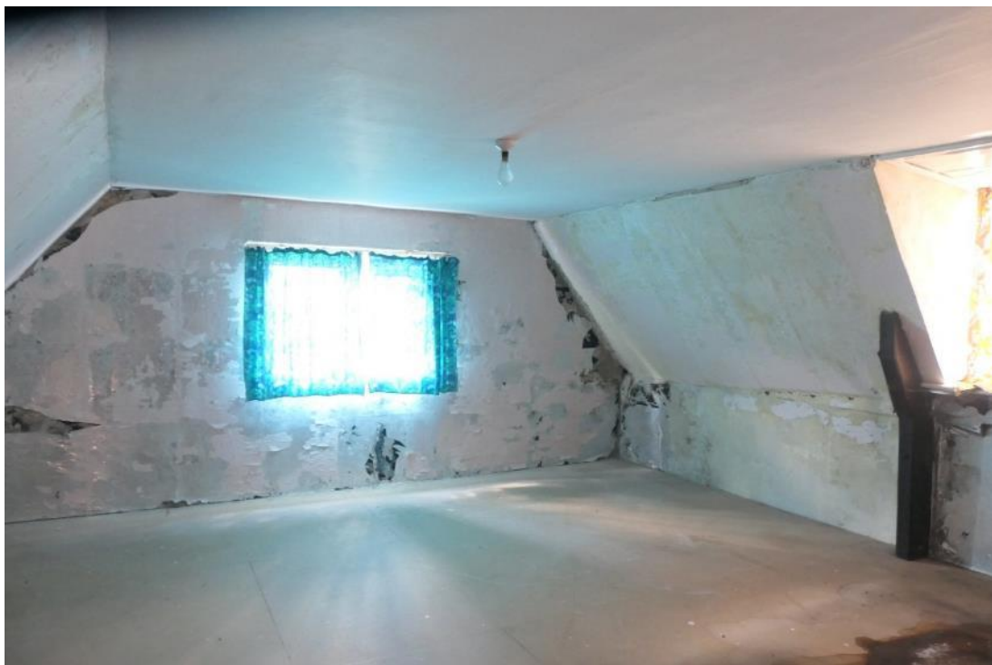
Photo 16 , internal view of the upper level of the main house.
