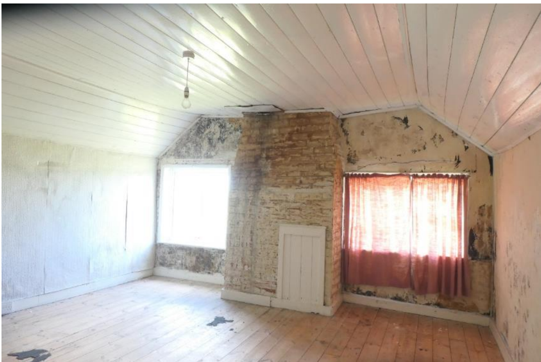
Photo 15 , internal view of the upper level of the northern extension.
