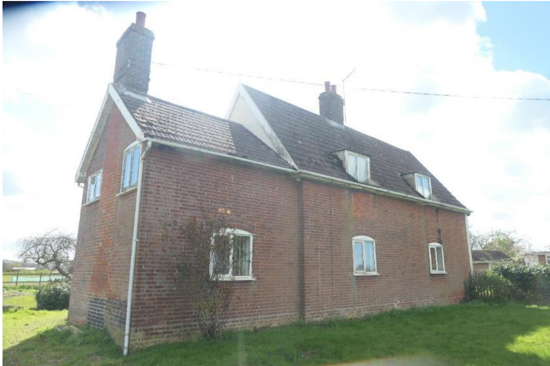
Photo 10 , north and west aspects of the building, looking southeast.
