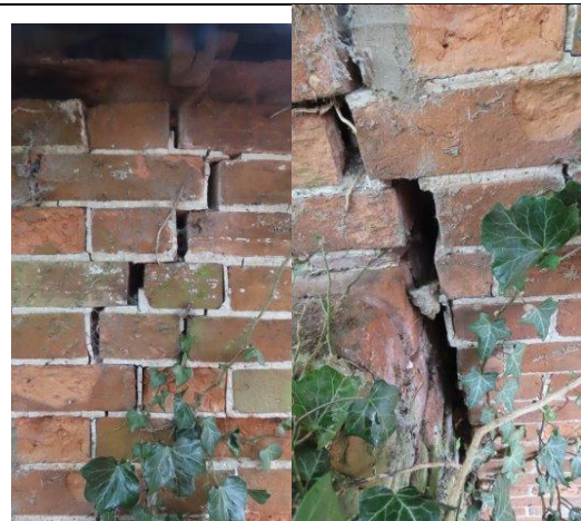
Subsidence and dislodged mortar on southern elevation.
