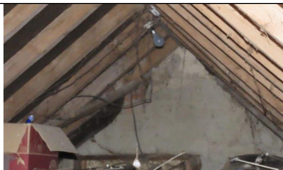
Roof void above workshop
