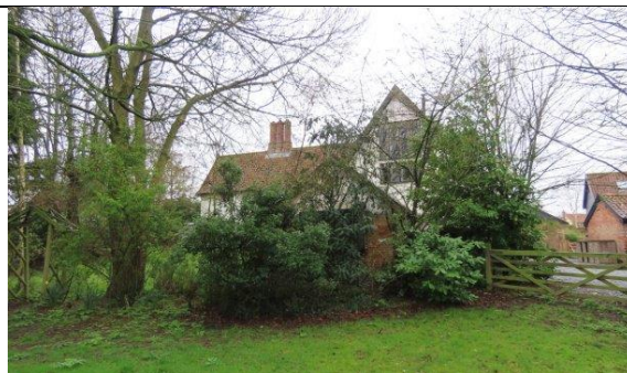
Northern elevation, showing ash tree to left and ornamental shrub covering northern elevation
