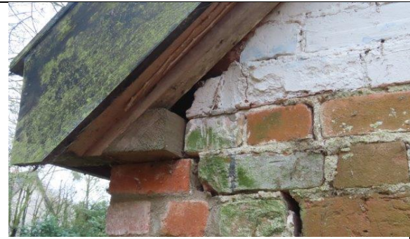
Subsidence and dislodged mortar on southern elevation.
