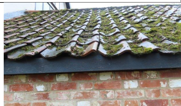
Lifted ridge tiles above eastern elevation
