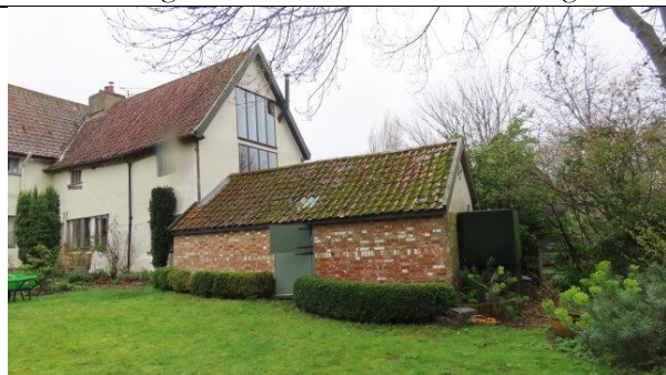
Eastern and western elevations of northern wing.
