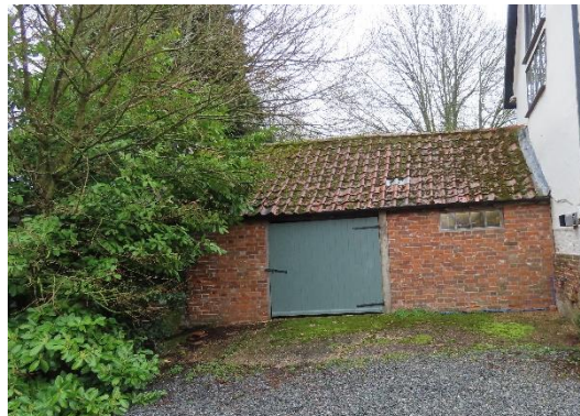
View of the western elevation of the northern extension
