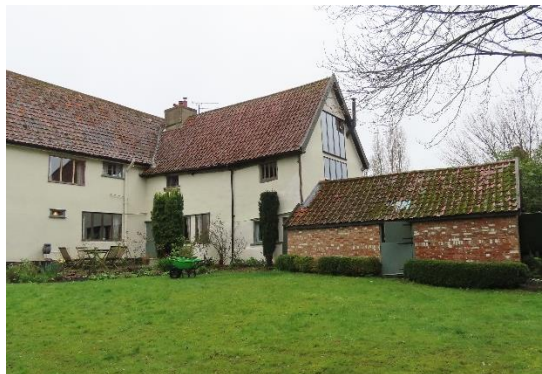
View of the eastern elevation of the northern extension
