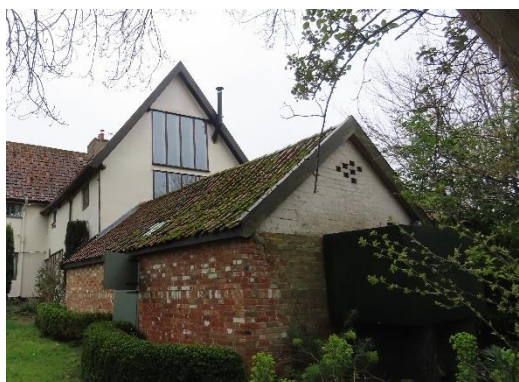
View of the northern and eastern elevations of the northern extension.
