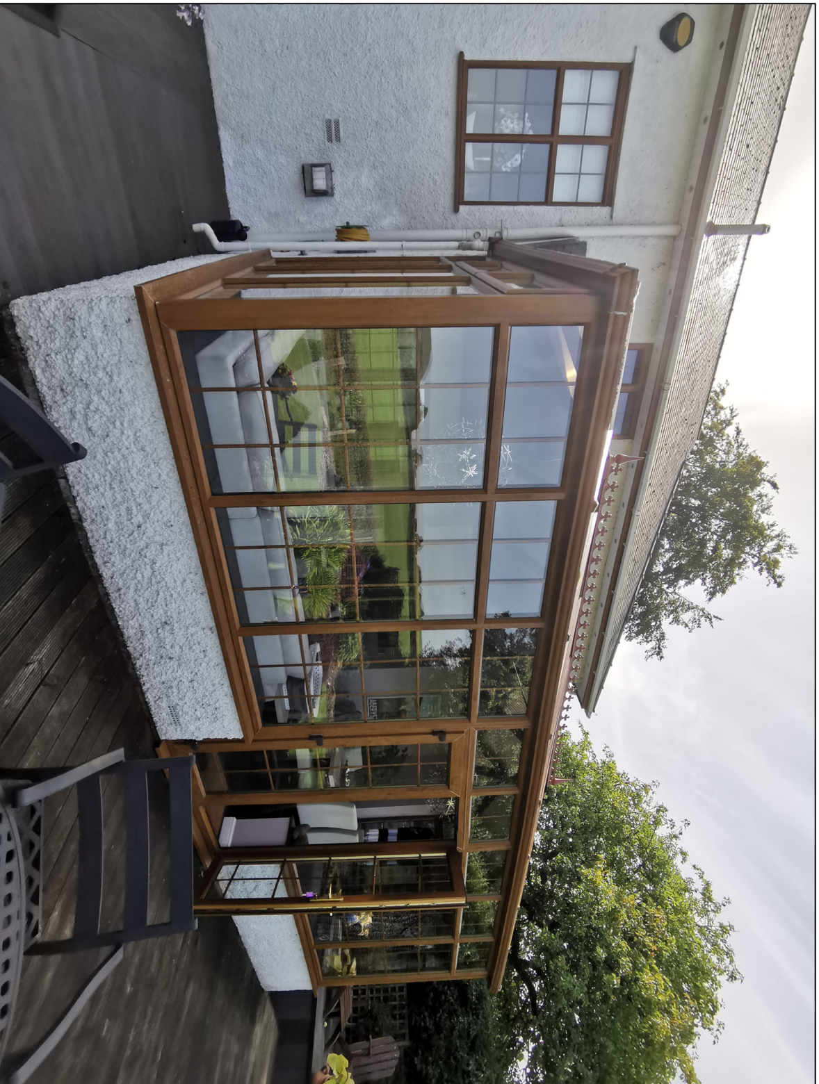
Existing Conservatory to be demolished
