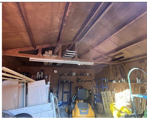
Photograph 6: Internal view of garage
