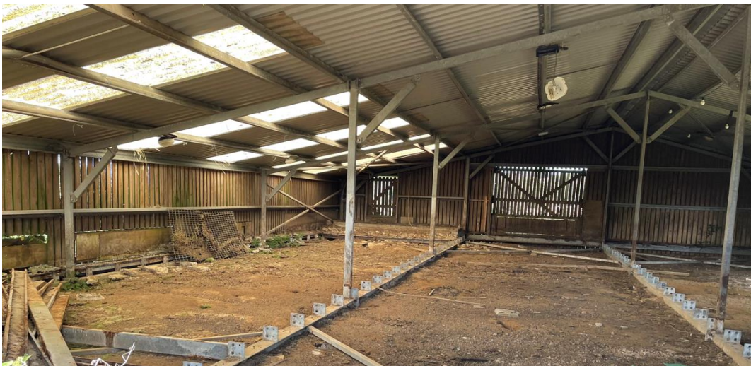
Interior of 'Barn 10'
