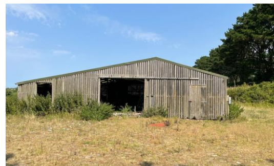
Former Duck Barn (Barn 10)
