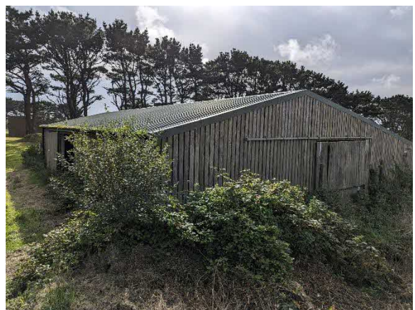
Photo 9. Showing Building E from the north
