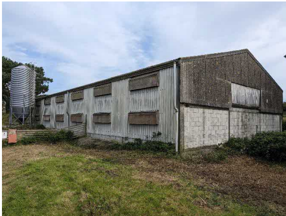
Photo 1. Showing Building A from the south west
