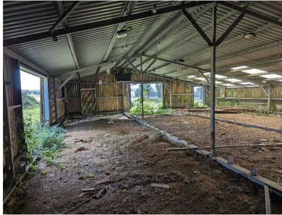
Photo 10. Showing the interior of Building E
