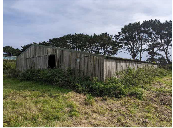
Photo 6. Showing Building C from the north
