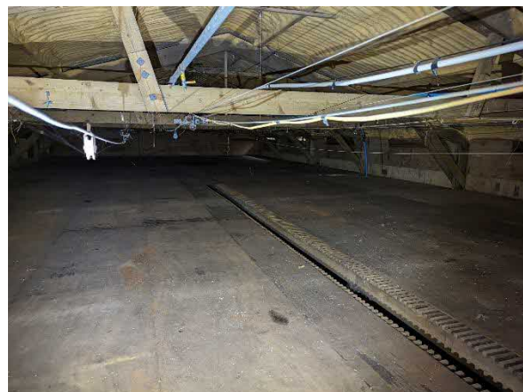
Photo 4. Showing the 1 st floor of Building A
