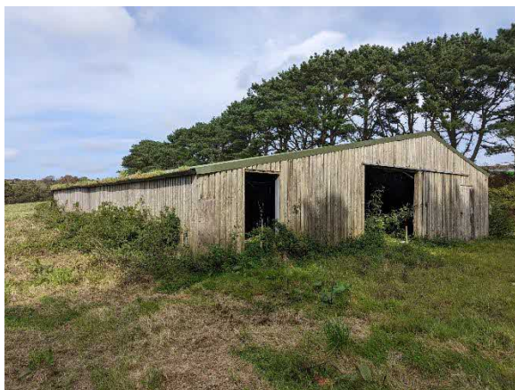
Photo 8. Showing Building E from the south
