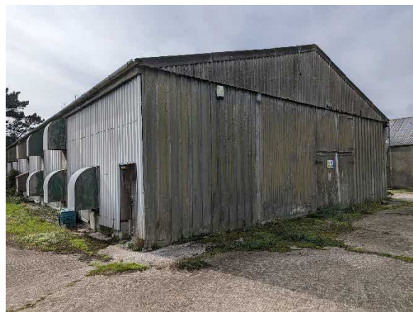
Photo 2. Showing Building A from the east
