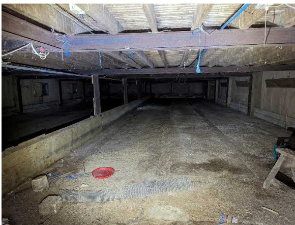
Photo 3. Showing the ground floor of Building A
