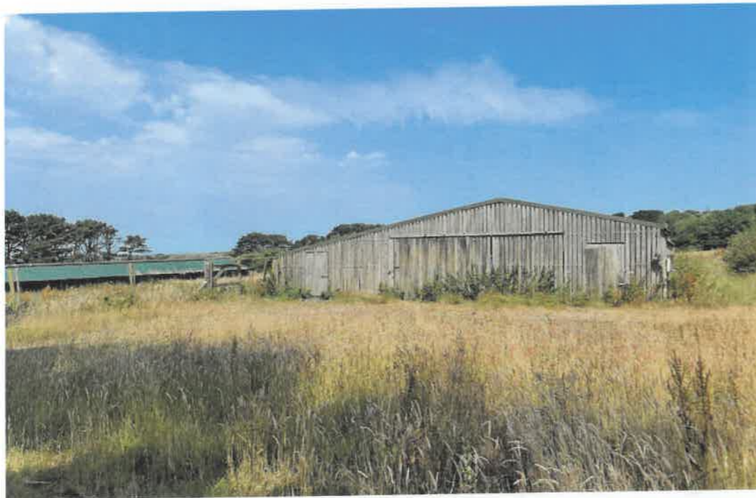
Photo 4 - South Elevation Barn 8
