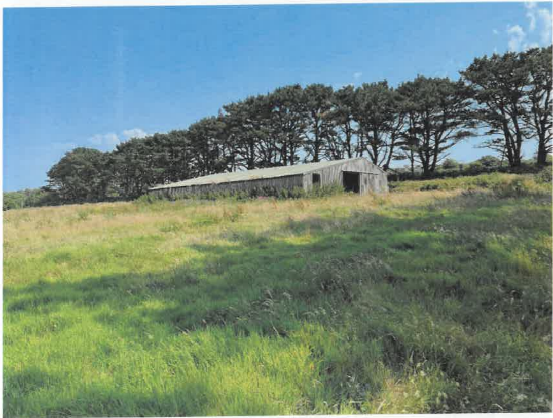
Photo 8 - West and South Elevations Barn 10
