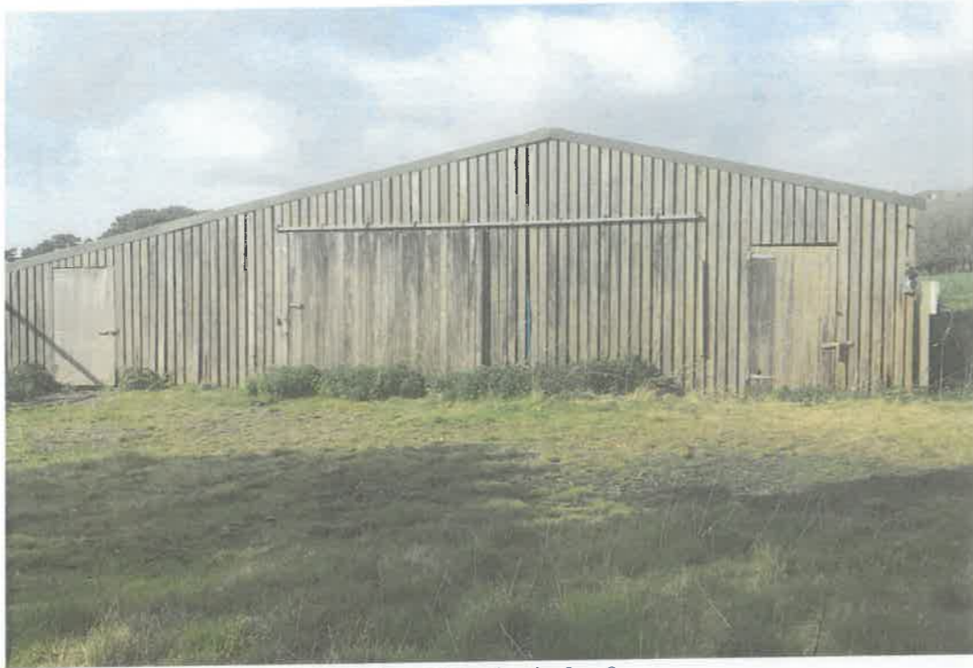
Photo 3 South Elevation Barn 8
