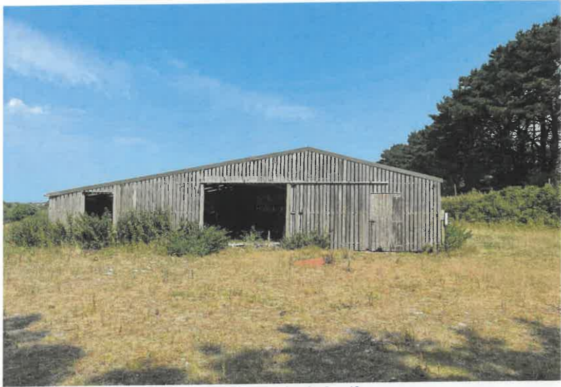
Photo 7 - South Elevation Barn 10
