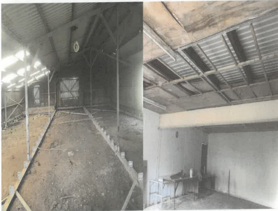
Photos 10-11 Typical View Showing Knee Brace Connection Rafter to Stanchion
