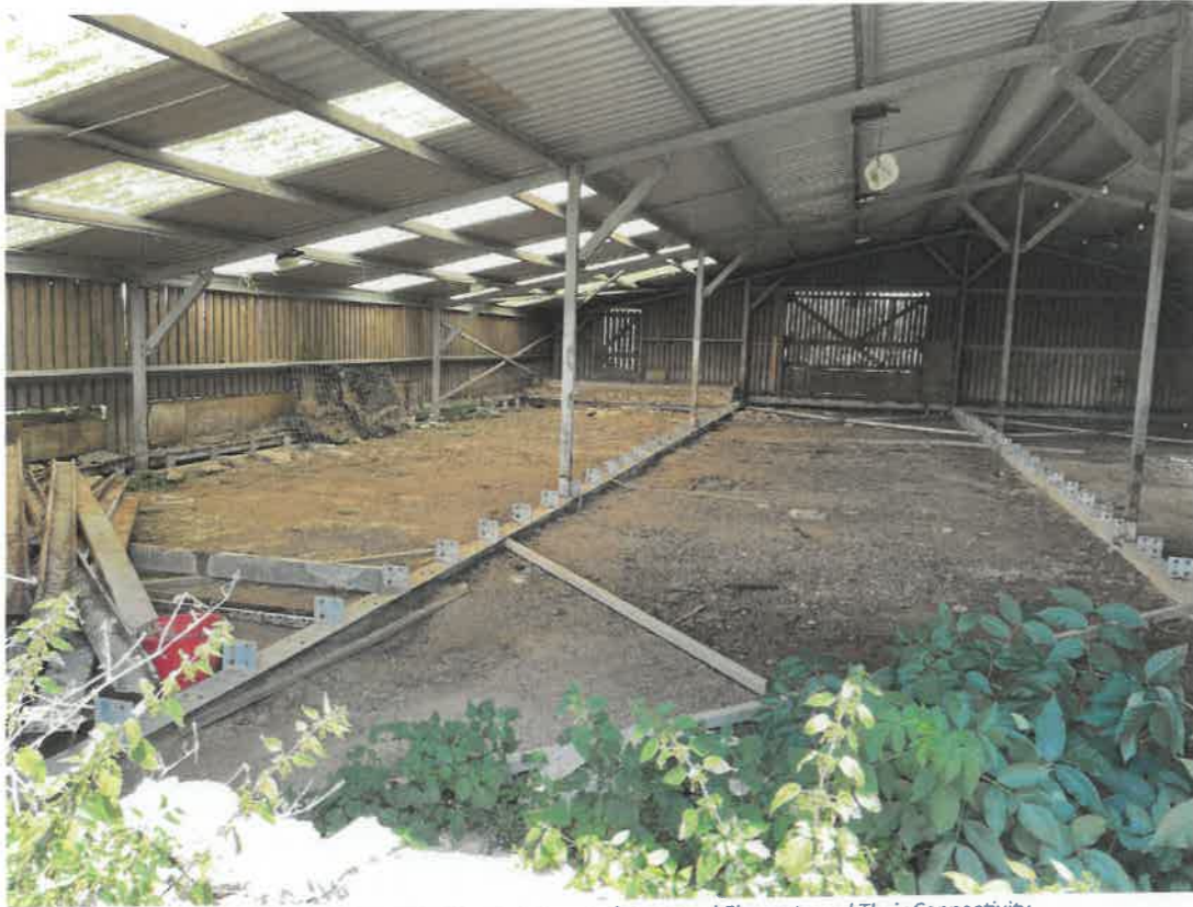
Photo 9 - Internal View Showing Full Range of Structural Elements and Their Connectivity
