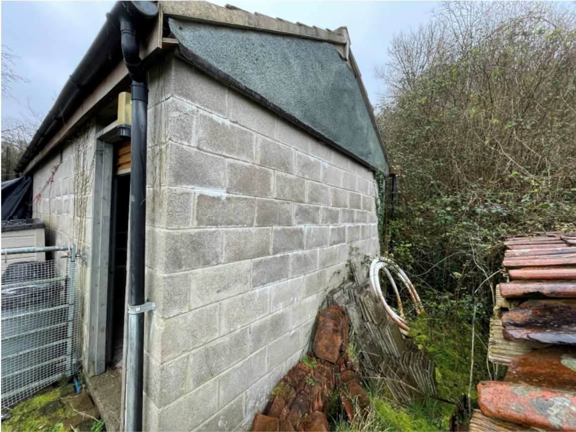
Photograph 5 – Outbuilding 1, from west
