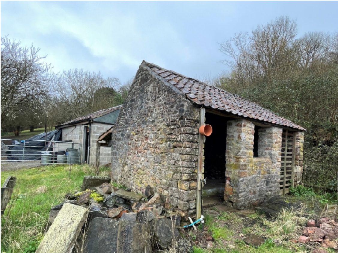
Photograph 2 – Outbuilding 2, from west
