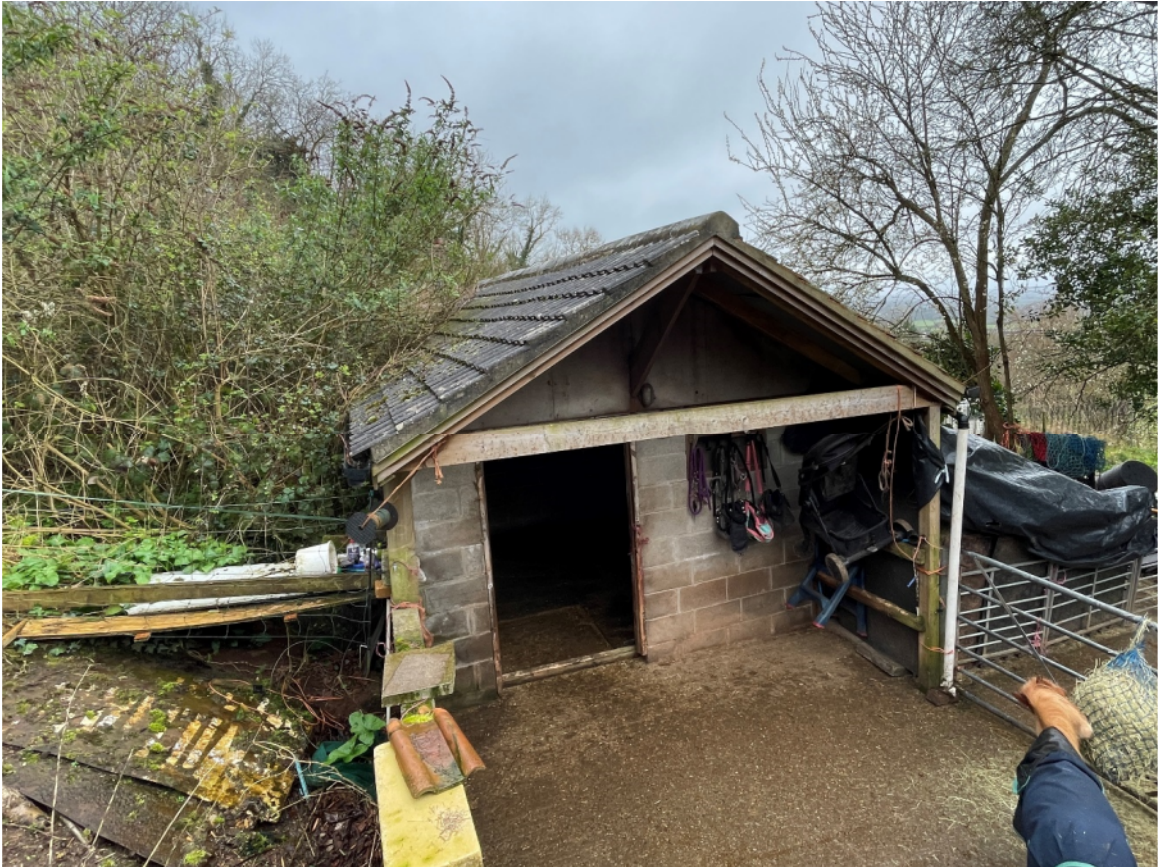
Photograph 6 – Outbuilding 1, from east
