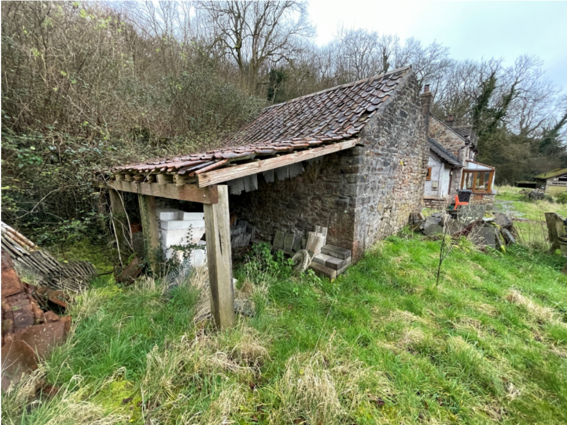
Photograph 3 – Outbuilding 2, lean-to from north-east
