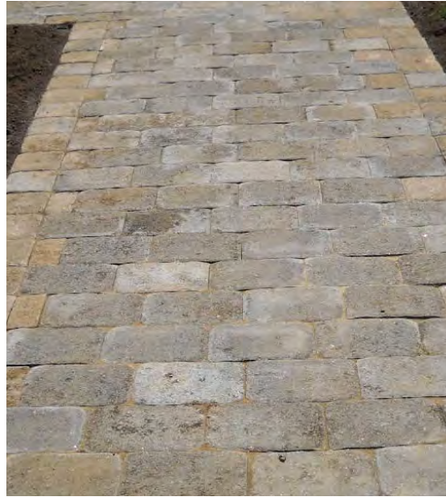
Buff brick paving
