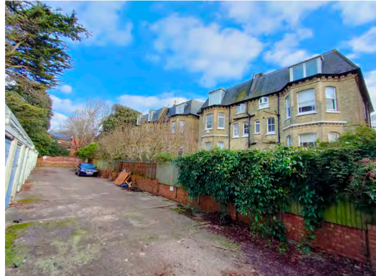
View north-east to rear of properties on Willbury Road
