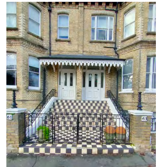
Ornate detailing on Willbury Road
