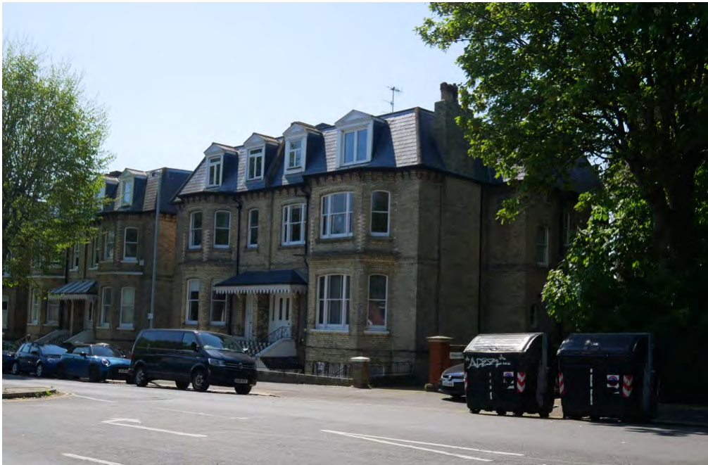
Figure 4 - Pair of Villa buildings (61- 63) to the south of the access to the garages.
