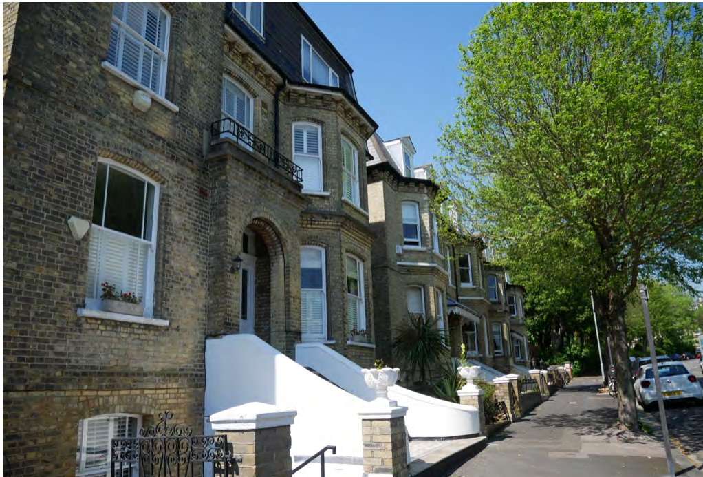
Figure 5 - View northwards along the line Villas
