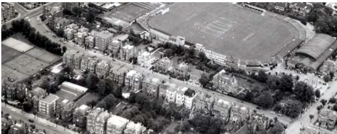
Figure 25 – The access can be seen turning to the rear behind the semi-detached pairs south of the tennis courts.
