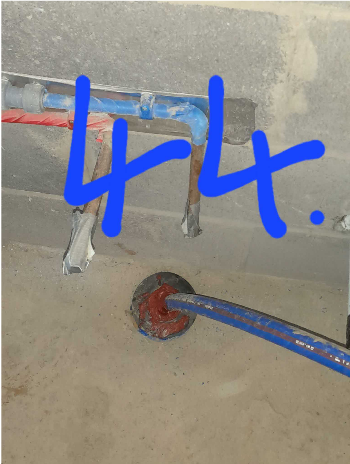
06 C8785E Plot 44 Internal service seal
