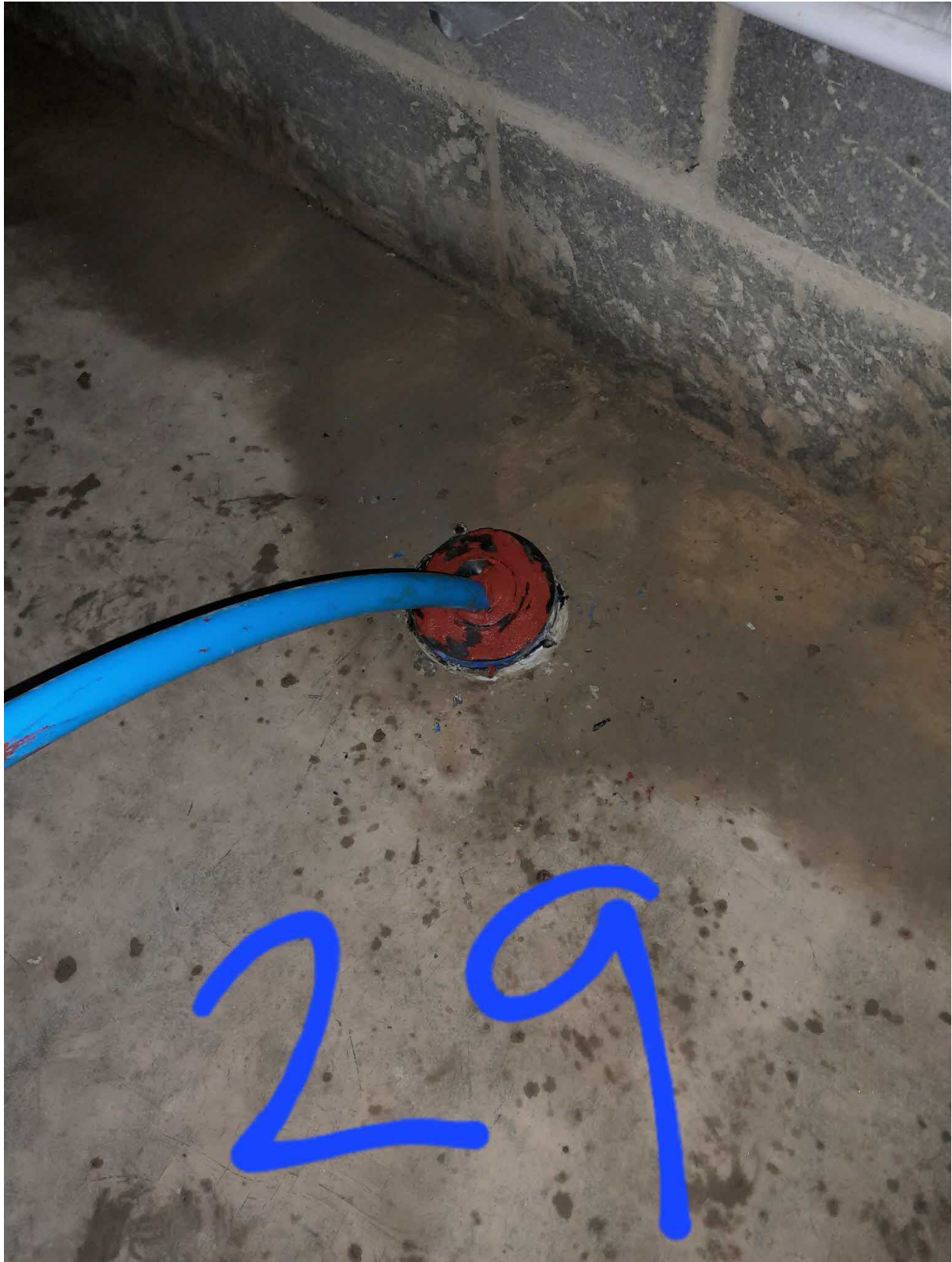
04C8785E Plot 29 Internal service seal
