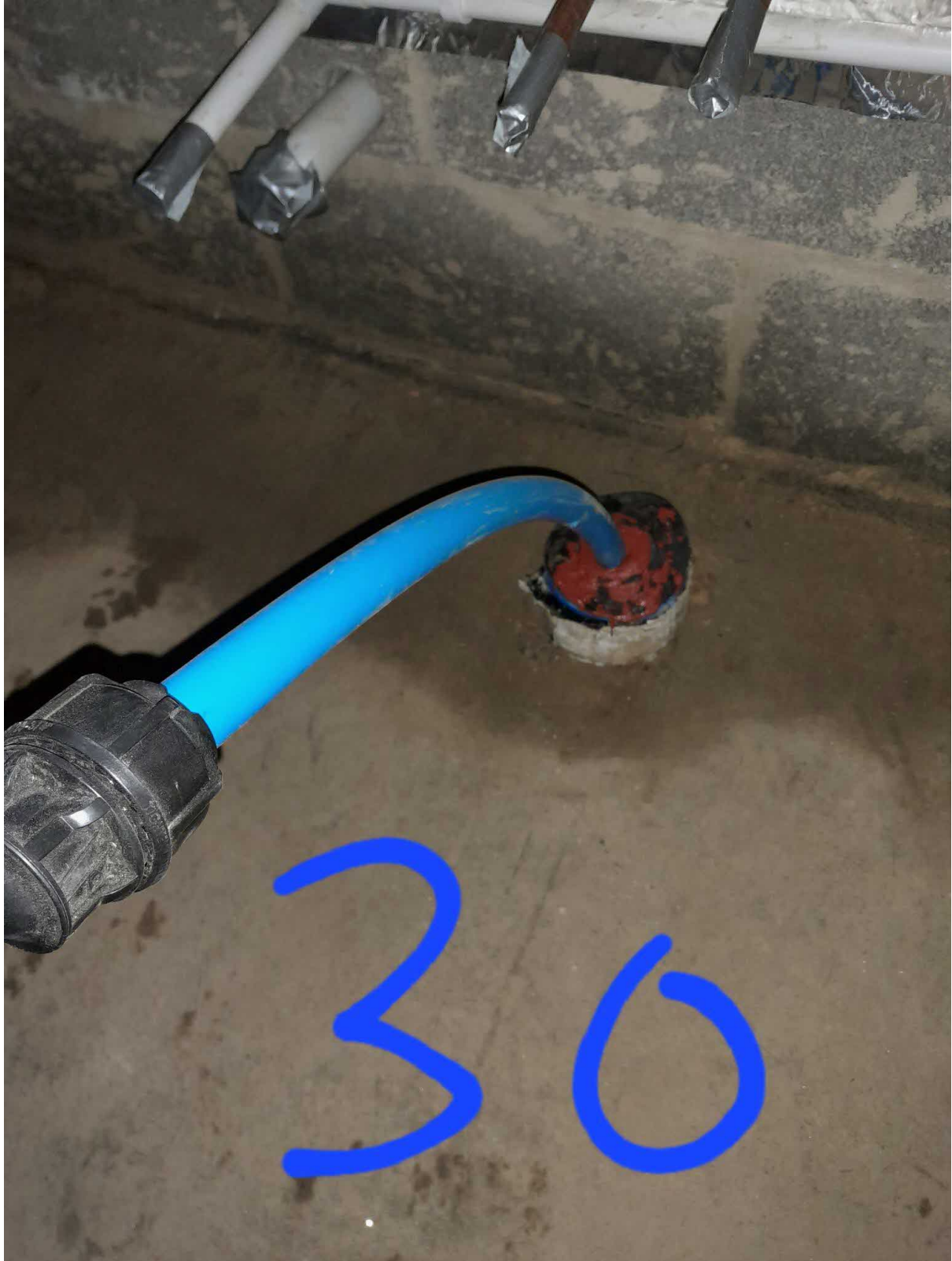
05 C8785E Plot 30 Internal service seal
