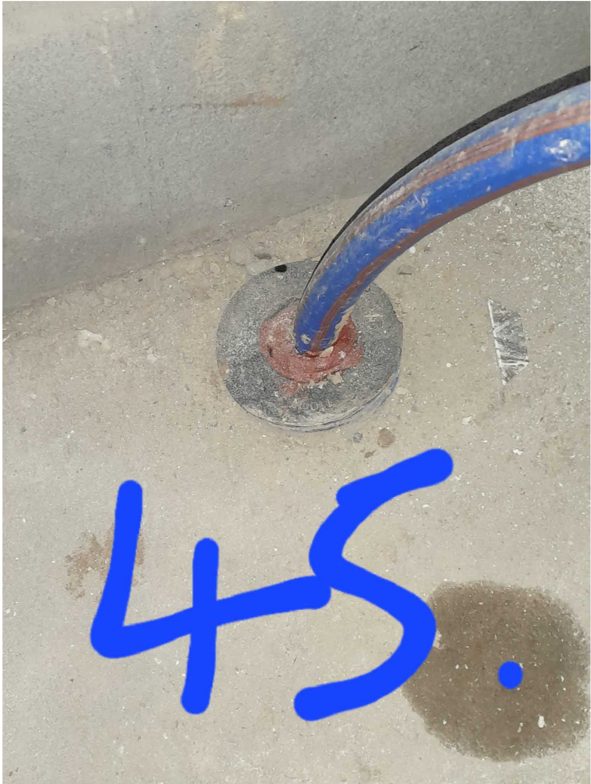
07 C8785E Plot 45 Internal service seal
