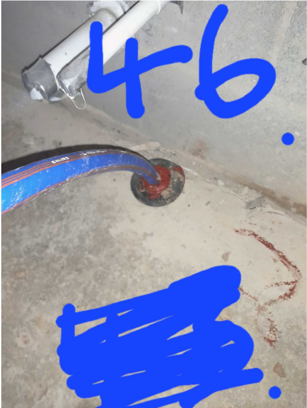
08 C87875 Plot 46 Internal service seal
