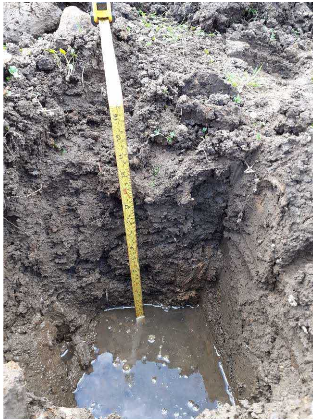
02 C8785E 18.03.24 Plot 21 Inspection pit
