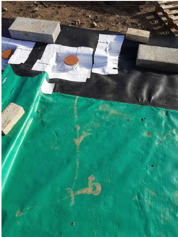
03 C8585E 29.09.22 Plot 51 Corners and Service Entry Duct
