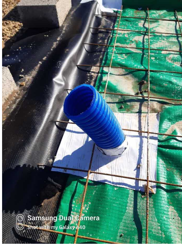
03 C8785E 03.04.23 Plot 52 Service Entry Duct (client photo)
