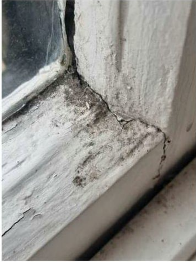
Tenon joints are splitting
