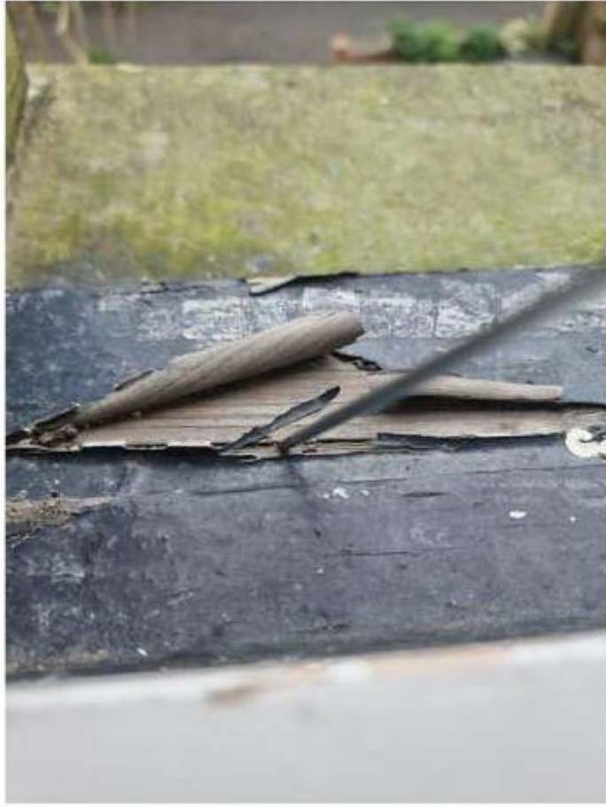
Rotting sill and tenon joint woodwork.
