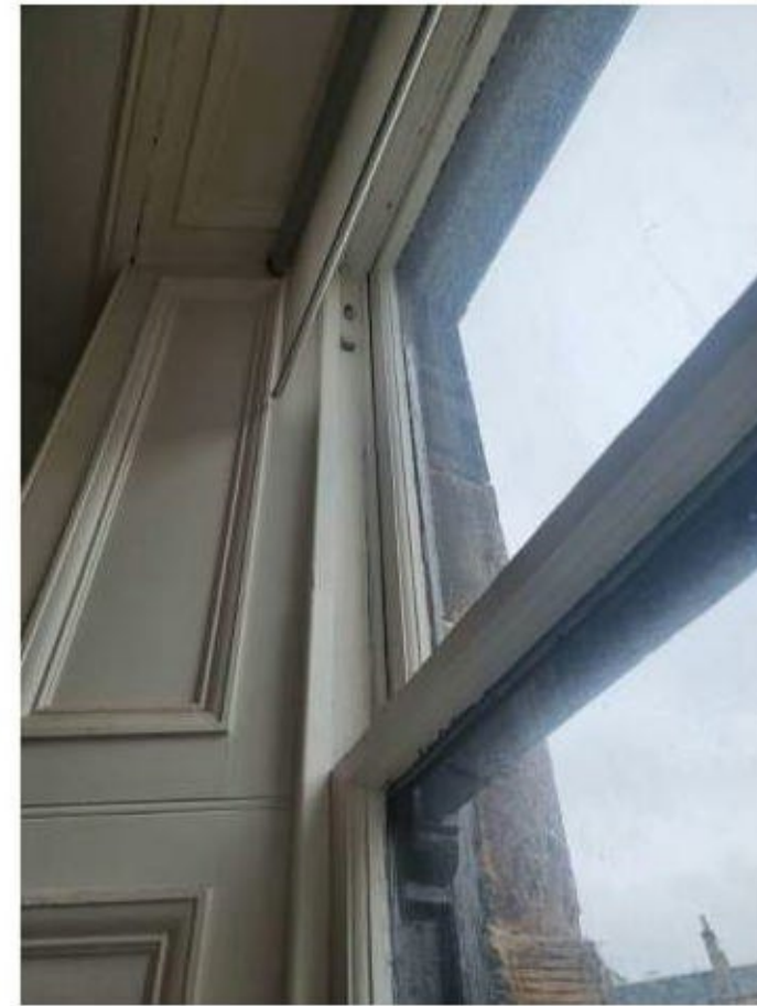
Mid rail woodwork is deteriorating. The second photo shows rope missing from another window.
