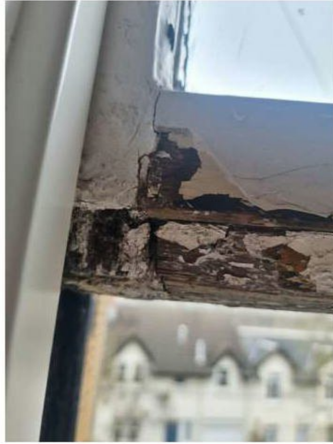
Rotting sill and tenon joint woodwork.
