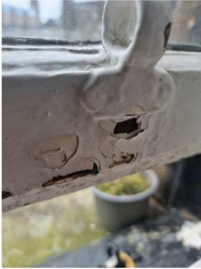
Rotting bottom rail woodwork.
