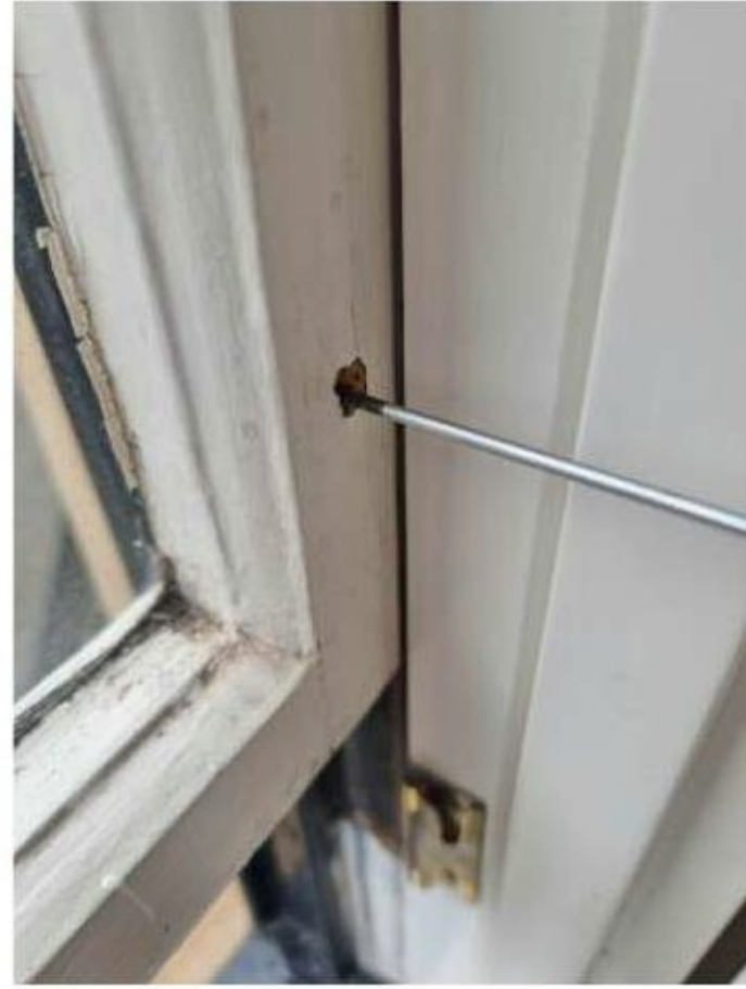
Rotting tenon joint and bottom sash.
