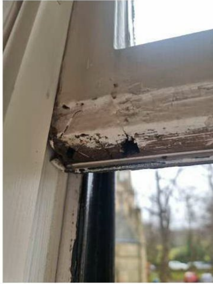
Rotting tenon joint and bottom sash.
