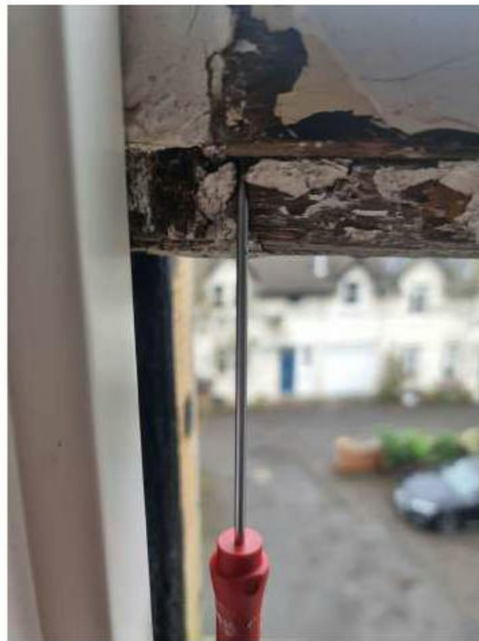
Rotting tenon joint and bottom rail.
