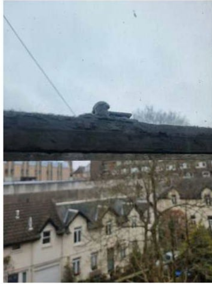
Rotting bottom rail and deteriorating mid-rail.
