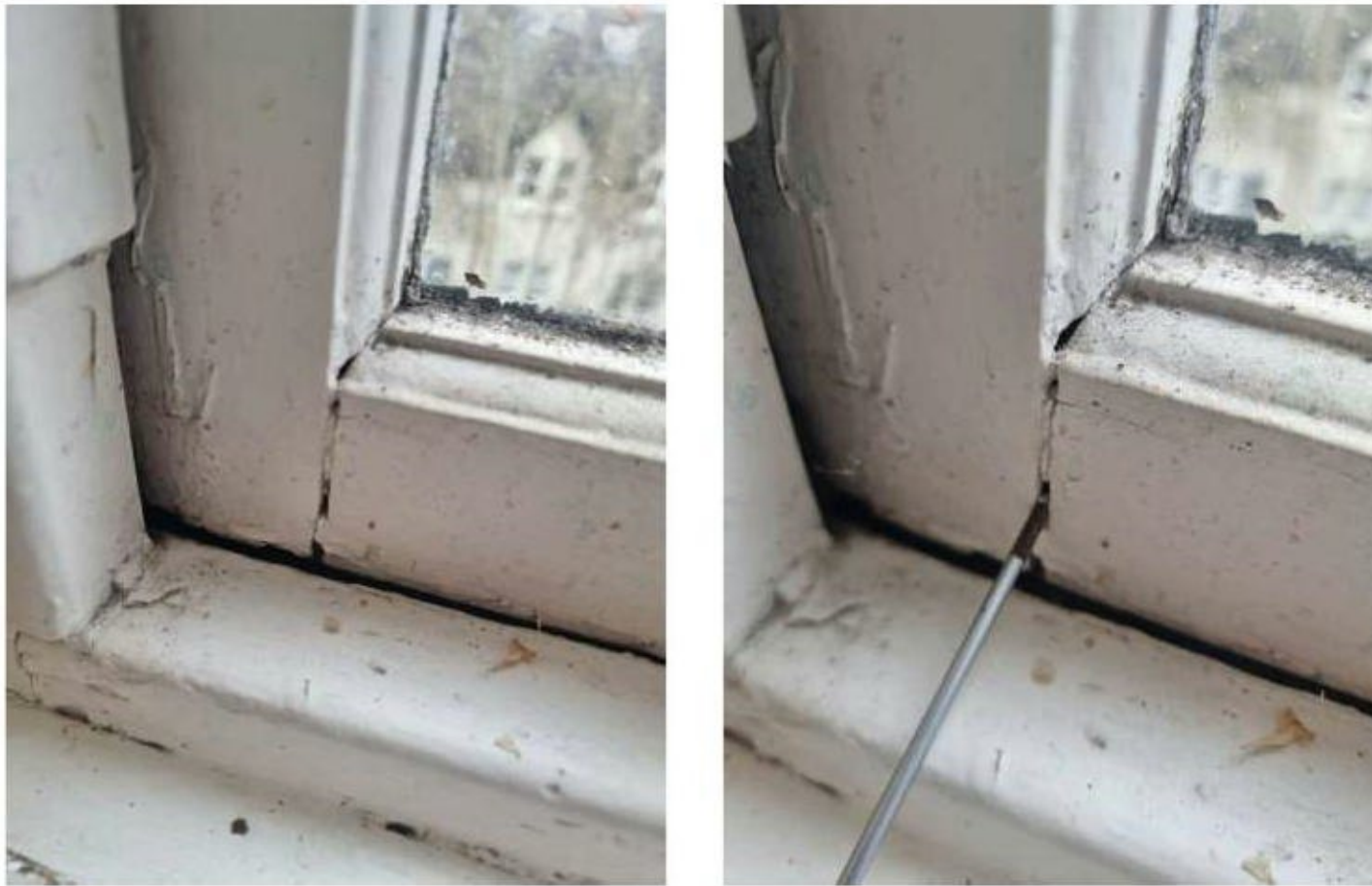
Splitting tenon joint with soft woodwork.
