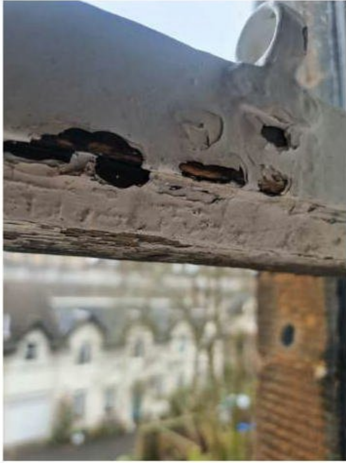
Rotting bottom rail and deteriorating mid-rail.
