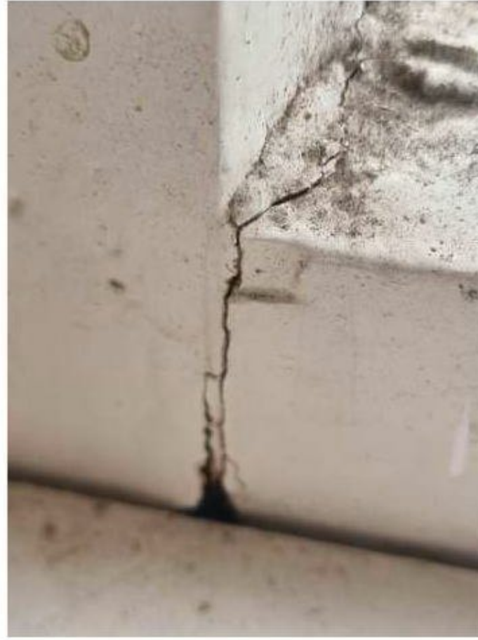
Tenon joints are splitting
