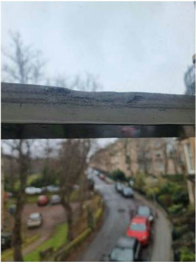
Mid rail woodwork is deteriorating. The second photo shows rope missing from another window.
