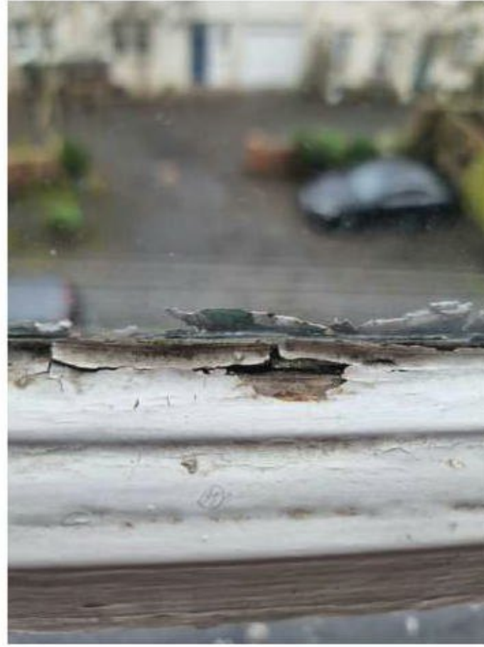
Rotting bottom rail woodwork.
