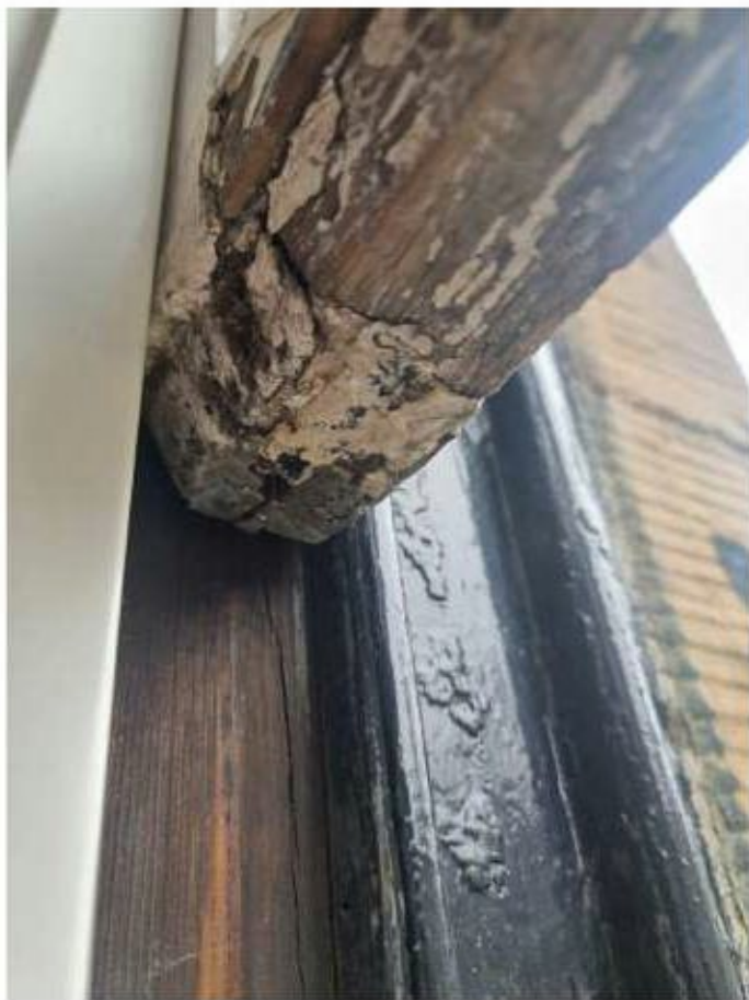
Rotting tenon joint and bottom rail.
