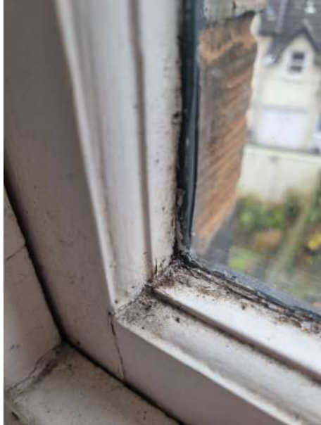
Seals are coming away from the glass which is allowing wind and water to enter the property. The second photo shows that the client is tying the bottom sash to the casement to stop the draught entering the property and the window rattling.
