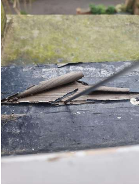
Rotting sill and tenon joint woodwork.
