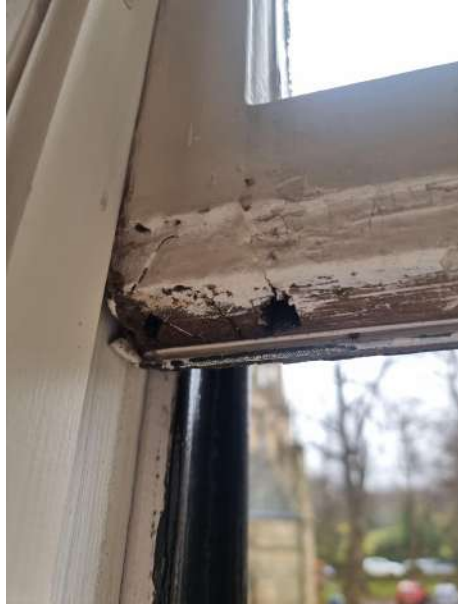
Rotting tenon joint and bottom sash.
