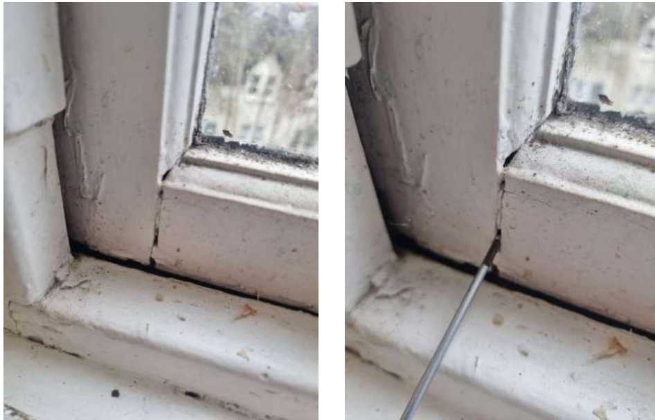
Splitting tenon joint with soft woodwork.
