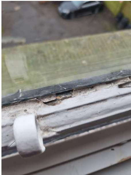
Seals and putty are coming away from the glass and deteriorating in areas. This is allowing water to penetrate the bare woodwork.
