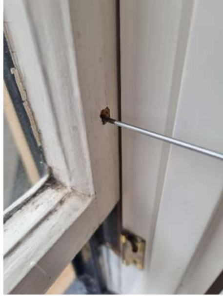
Rotting tenon joint and bottom sash.
