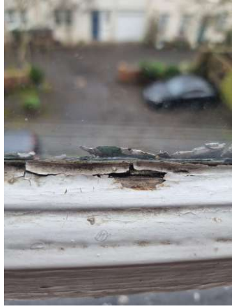
Rotting bottom rail woodwork.
