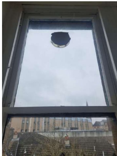
Window is badly out of alignment which is furthering the issue with wind and water entering the property. The second photo is of a fan in the window which would be removed when replacing the windows.
