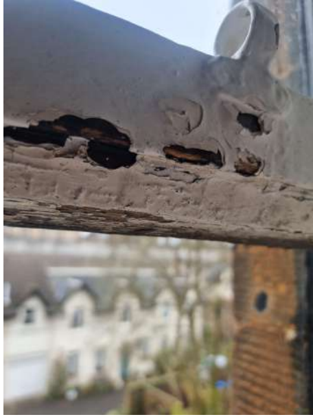
Rotting bottom rail and deteriorating mid-rail.
