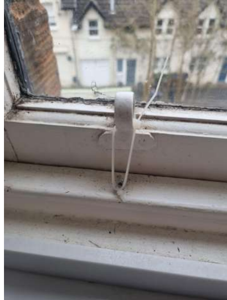
Seals are coming away from the glass which is allowing wind and water to enter the property. The second photo shows that the client is tying the bottom sash to the casement to stop the draught entering the property and the window rattling.
