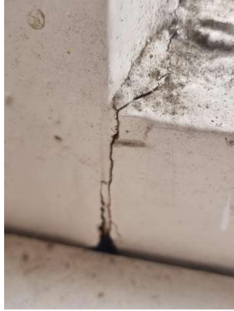
Tenon joints are splitting
