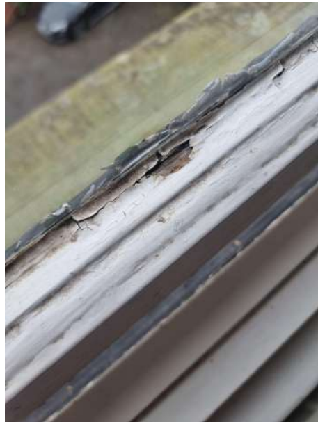
Seals and putty are coming away from the glass and deteriorating in areas. This is allowing water to penetrate the bare woodwork.
