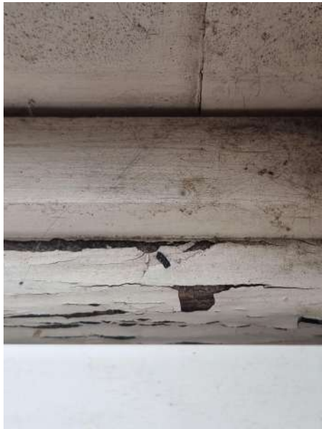
Internal wood is bare and showing signs of rotting. Rope is missing from a few windows and therefore they are non-operational.
