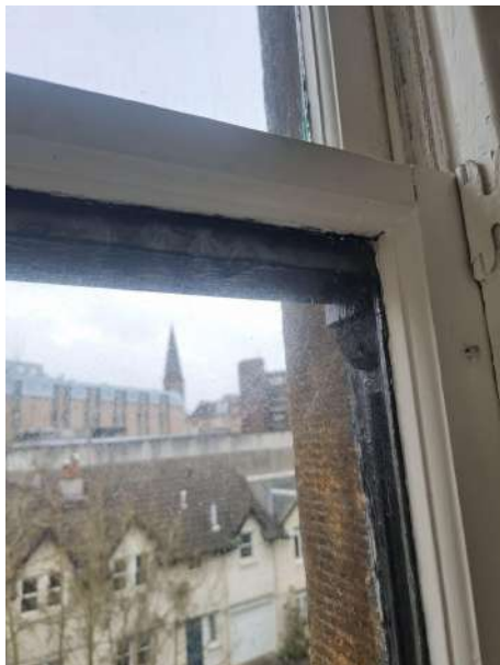
Window is badly out of alignment which is furthering the issue with wind and water entering the property. The second photo is of a fan in the window which would be removed when replacing the windows.
