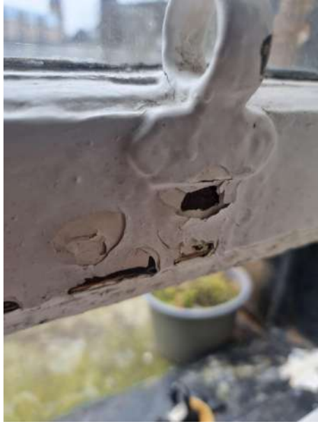
Rotting bottom rail woodwork.
