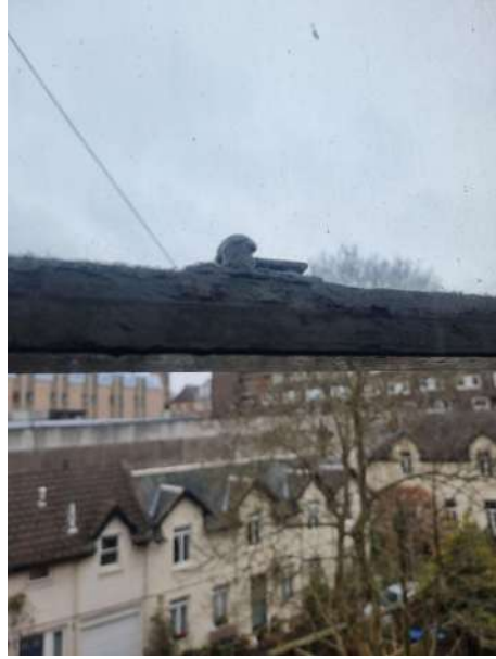
Rotting bottom rail and deteriorating mid-rail.
