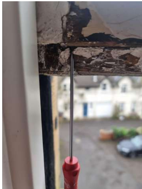
Rotting tenon joint and bottom rail.
