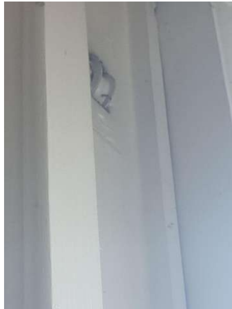
Internal wood is bare and showing signs of rotting. Rope is missing from a few windows and therefore they are non-operational.
