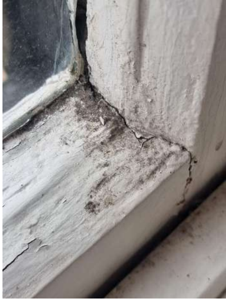
Tenon joints are splitting
