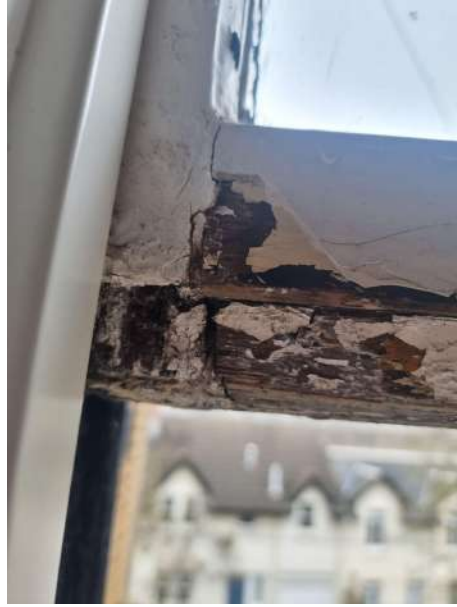
Rotting sill and tenon joint woodwork.
