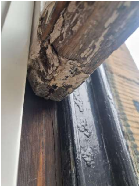
Rotting tenon joint and bottom rail.
