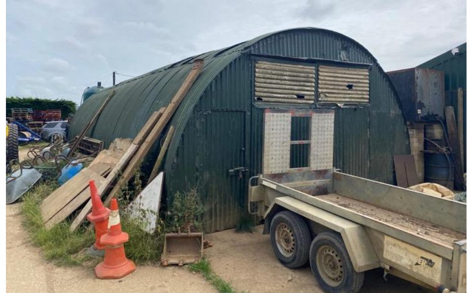
Image 4 – existing building no 2
