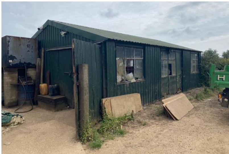
Image 3 - Existing building no 1
