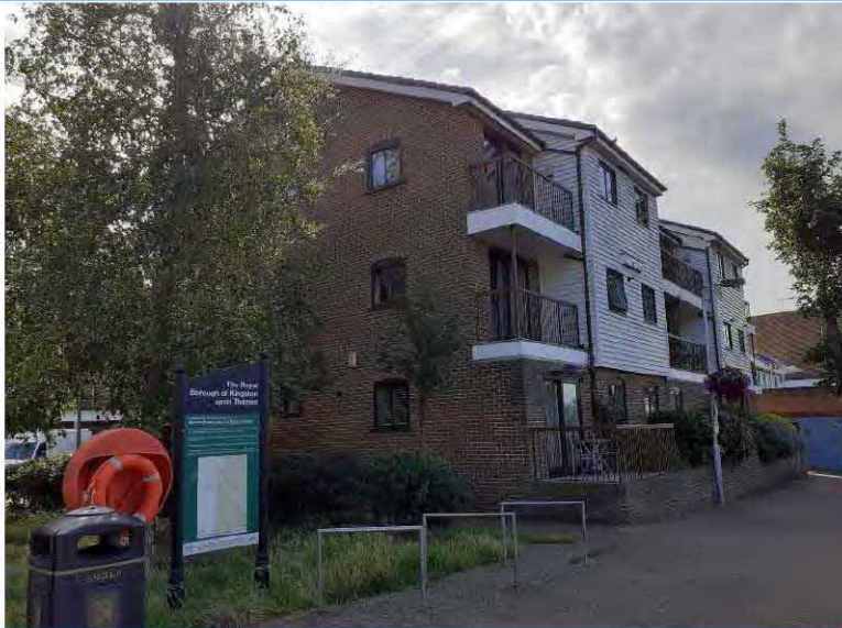
13 – Flats adjacent to southern boundary, looking south
