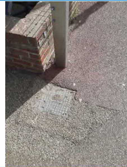
32 – Service cover adjacent to northern boundary, looking east
