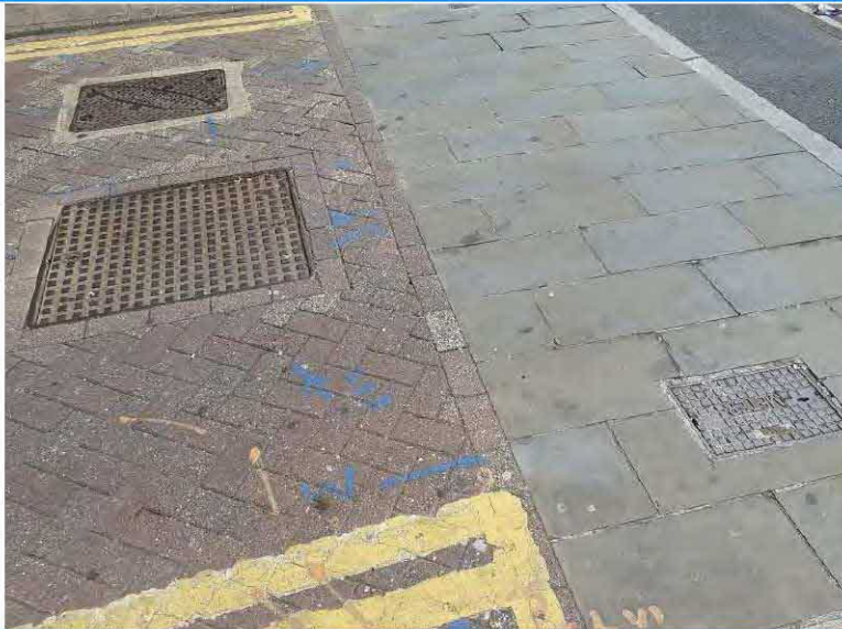
37 – Service covers at site entrance, looking north
