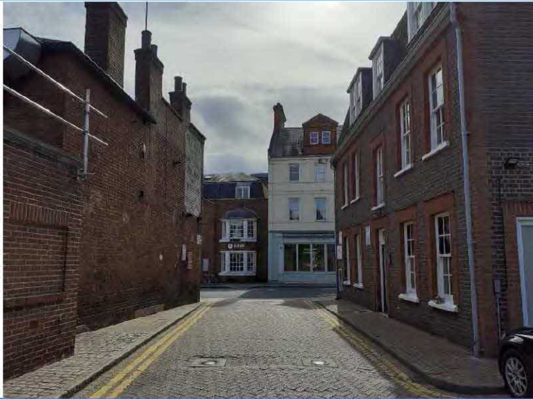
5 – Looking east along Ram Passage
