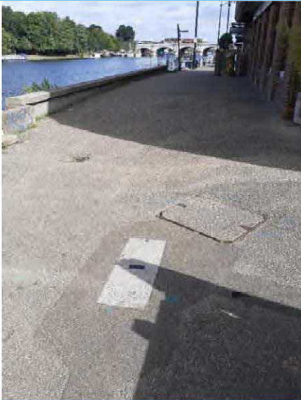
33 – Service covers, looking north along footpath
